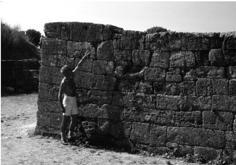
Fig. 11.5 The author inspecting the walls of ancient Troy built out of the local bedrock limestone (Rapp 1982)
