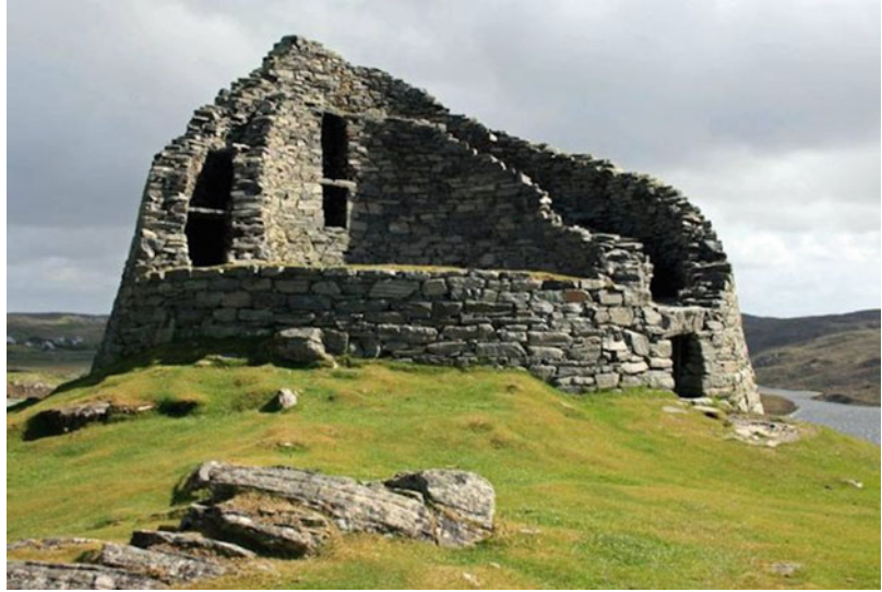
Fig. 6.2 Dimension stone. Middle Jurassic sandstones. Dun Beag Broch, west coast of the Isle of Skye, Scotland. Historic Scotland
