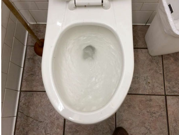
Fig. 7.8 Keeping it clean – flushing a cistern
