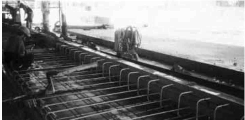
Figure 6-1 Ledged spandrel in form.
