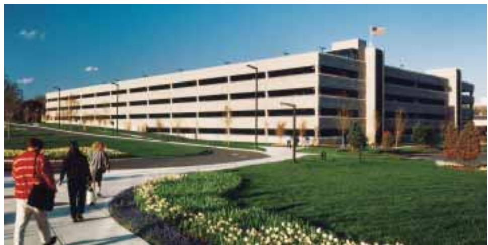
Pfizer Inc. Parking Structure (Building 290), Groton, CT
