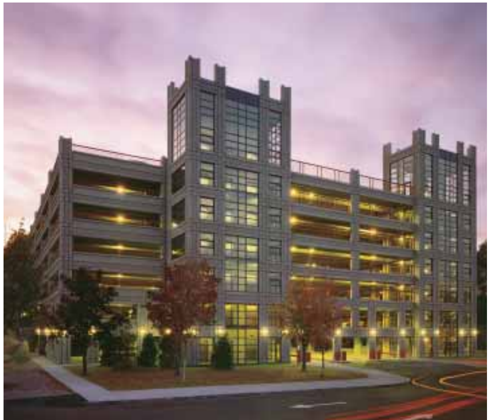
Boston College Parking Structure, Chestnut Hill, MA
