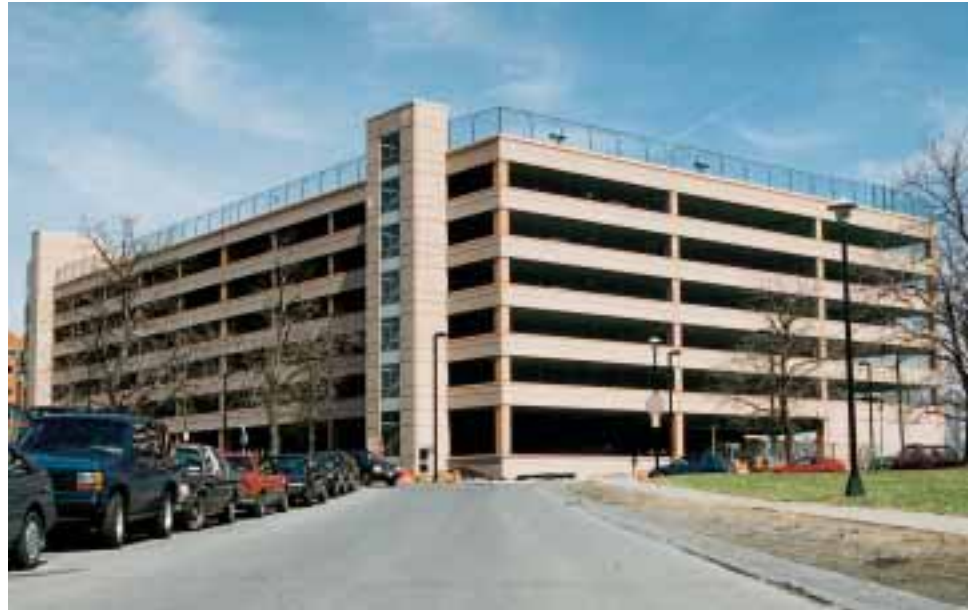
Albany Medical Center Parking Structure, Albany, NY
