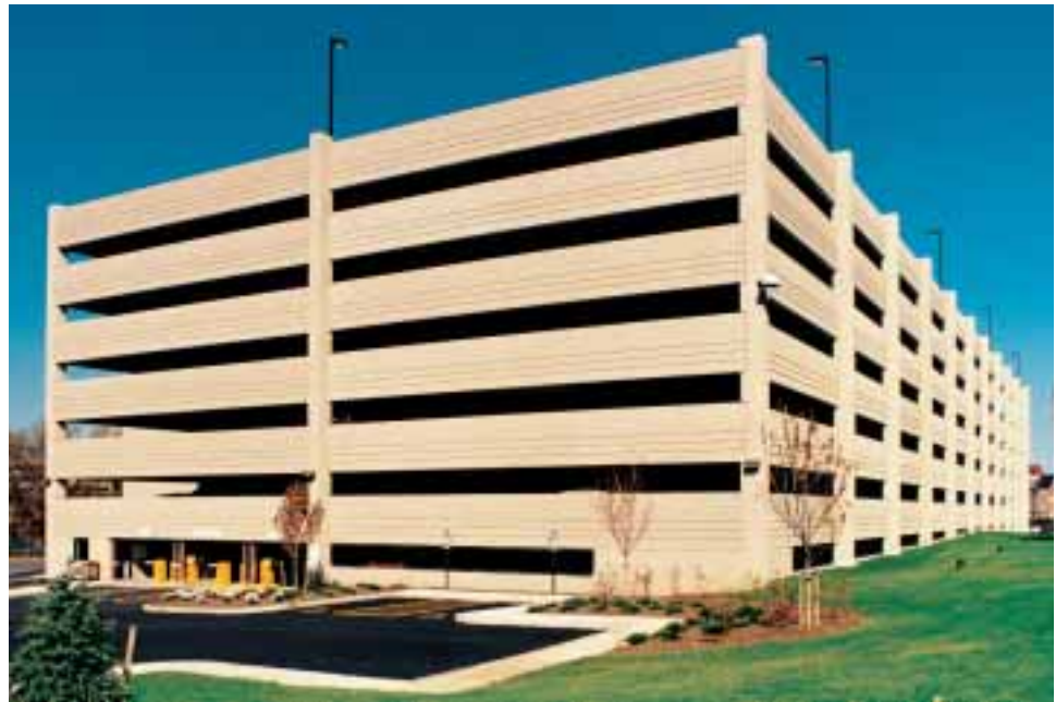
Station Plaza Parking Garage, Trenton, NJ
