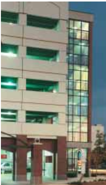
Carriage Park Parking Garage, Lincoln, NE
