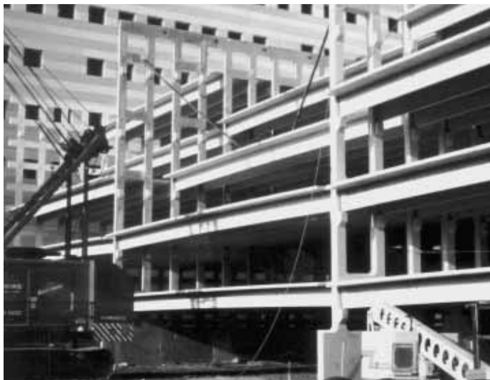
Figure 7-3 Braced “lite walls” during erection.
