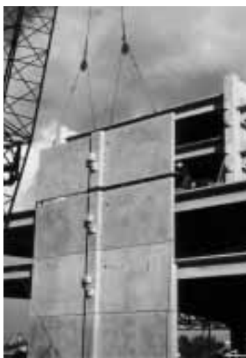
Figure 7-4 Story height wall panels “Stacked.”
