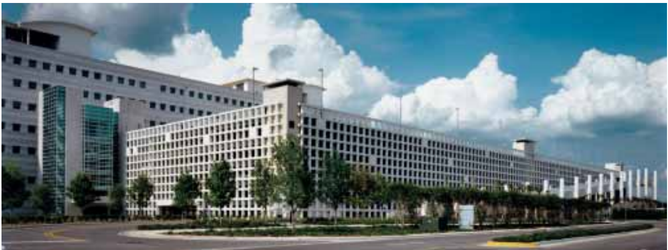
USAA Southeast Regional Office Parking Structure, Tampa, FL
