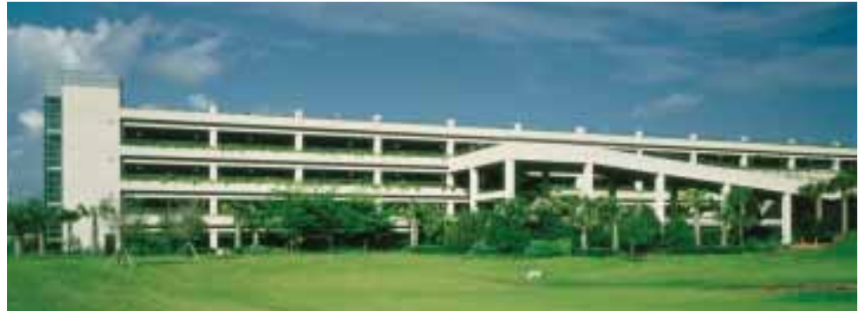
Kravis Center Parking Structure, West Palm Beach, FL
