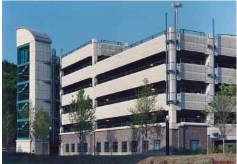
Pittsburg Technology Center Garage, Pittsburg, PA
