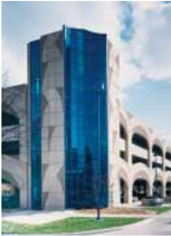
Chauncey Swan Plaza Parking Facility, Iowa City, IA
