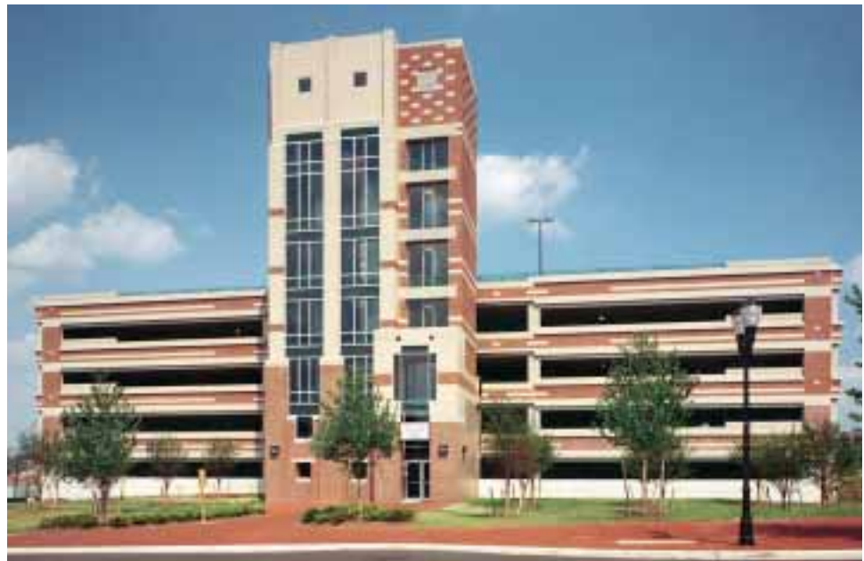
Camden Waterfront Parking Garage, Camden, NJ
