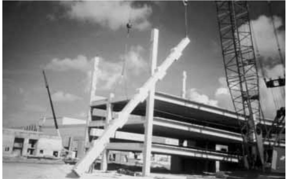
Figure 7-2 Rotating a column into position.
