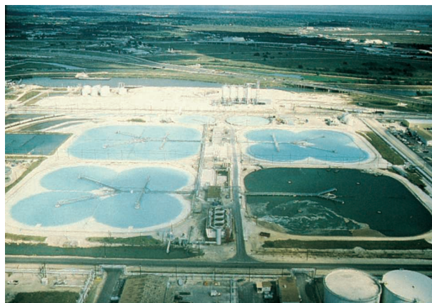
Magnesium hydroxide was precipitated from processed seawater in settling ponds at the Dow Chemical Company once operated in Freeport, Texas.
