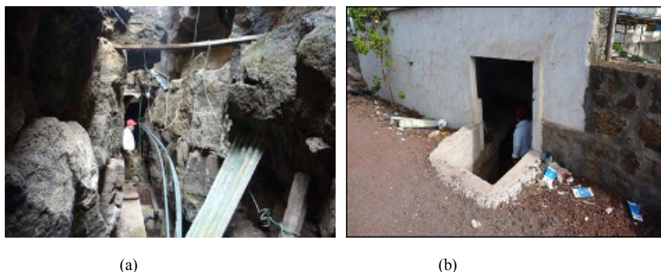
Figure 3.1-Pictures of (a) different pipes and b) entrance of Misión Franciscana Crevice.
