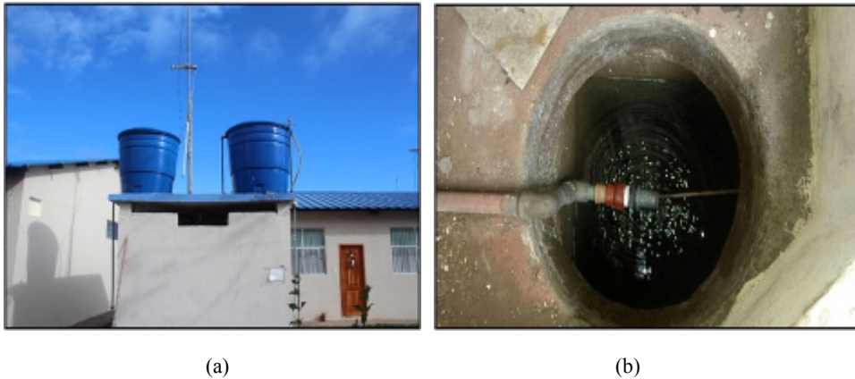
Figure 4.2- Typical (a) elevated tank and (b) cistern in Puerto Ayora.
