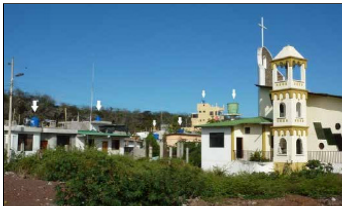
Figure 3.6- Picture showing several elevated tanks within Puerto Ayora.
