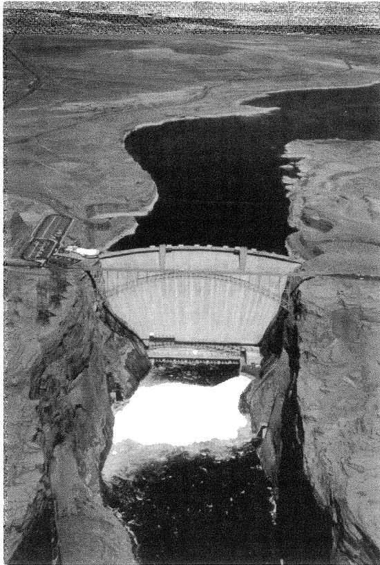
Figure 6.1 Glen Canyon Dam in March 1996, showing experimental discharge of 45,000 cubic meters per second. The experiment is an attempt to recreate primeval ecology of the Colorado River as it passes through the upper portion of the Grand Canyon in Arizona.
