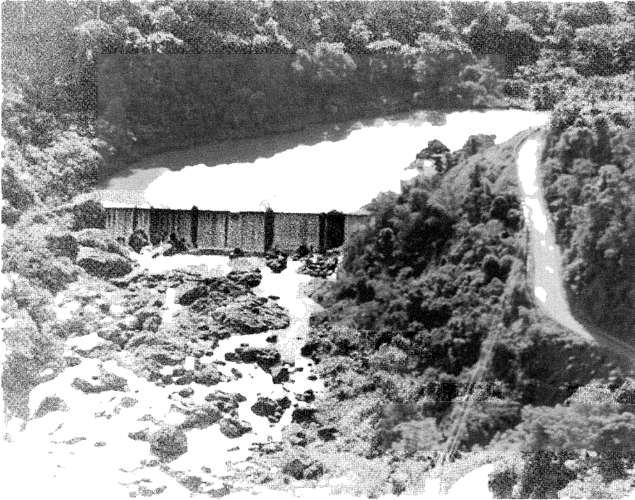
Figure 4.12 The small Comerio 1 reservoir on the La Plata River was abandoned long ago as a public water supply source due to sewage contamination from the town of Comerio. (Photo by Guillermo Sosa.)
