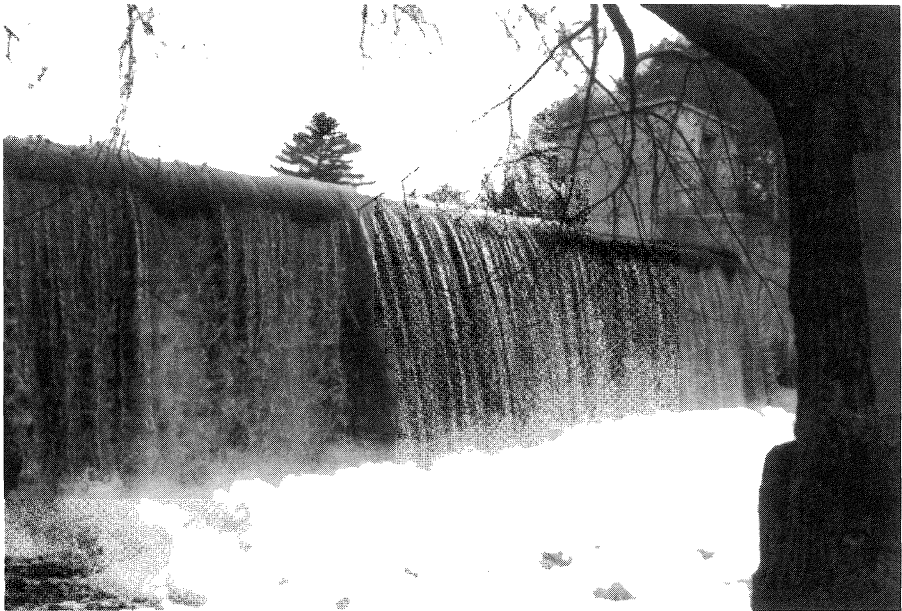
Figure 3.49 Spillway of Norton Reservoir Dam on Rumford River.
