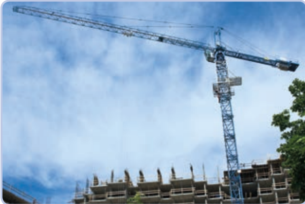
Figure 11-48: A real tower crane at work. As you can see, its tower mast is built with a Brown truss, and its jib is built with a triangular Warren truss, just like in our model.
