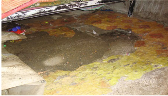
Fig. 6.2 A sinking floor due to the absence of steel support and movement of the soil.
