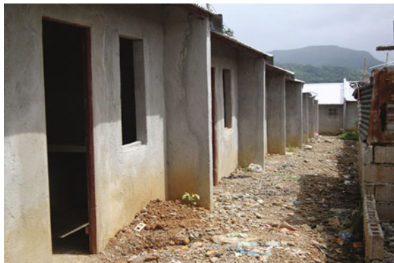
Fig. 6.1 Some of the unfinished and unoccupied housing units in Southville Rodriguez Housing Project (SRHP) Phase 8A. Source Author
