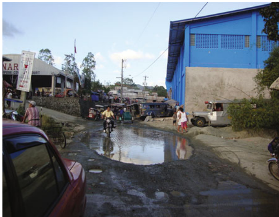
Fig. 5.5 The rough road at the main entrance of the SRHP. Source Author
