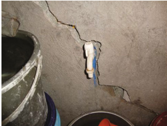
Fig. 6.3 A cracked bathroom wall caused by gradual movement of the ground.
