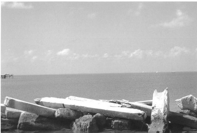
FIGURE 7.3 Photo of a manmade jetty in Palm Beach. Rock jetties and breakwaters are common on many beaches. They are designed and engineered to reduce erosion and they are the source of many serious accidents.
