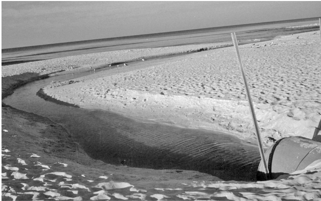
FIGURE 7.7 Open outfall stretching across Panama City Beach. Outfalls are often the source of pollution and consequently represent a hazard, especially to children.
