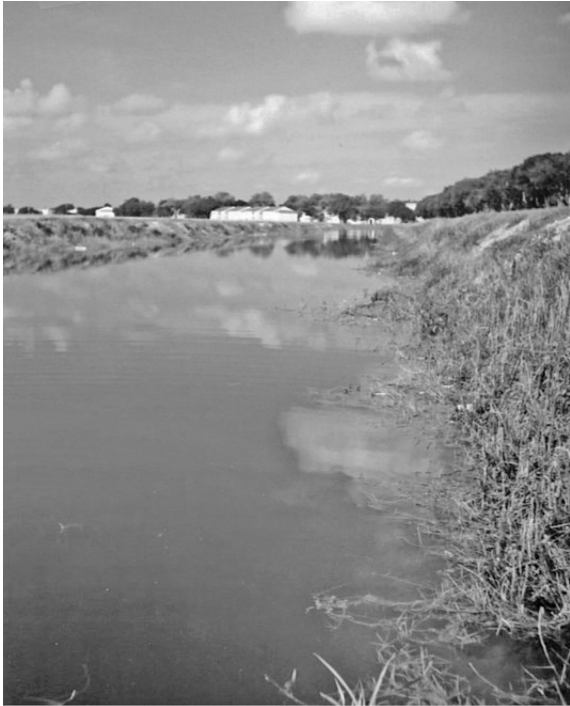
FIGURE 7.24 Typical canal with steep embankment leading directly to deep water.
