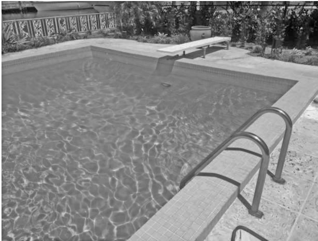
FIGURE 6.12 A backyard pool with no depth markings, no bottom markings, and no posted rules.
