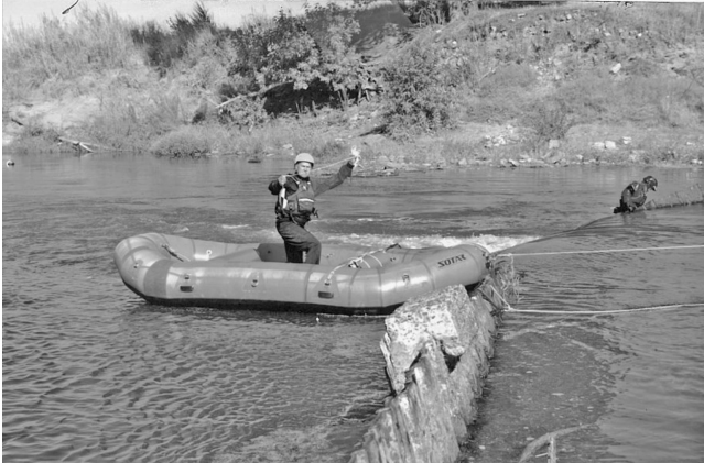
FIGURE 14.5 Low-head dams are often responsible for creating hydraulic currents, which have been responsible for more than 100 drownings.
