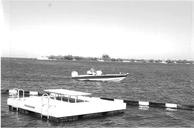
FIGURE 7.6 Floating docks designed for recreation should be anchored in deep water to prevent a diving injury.
