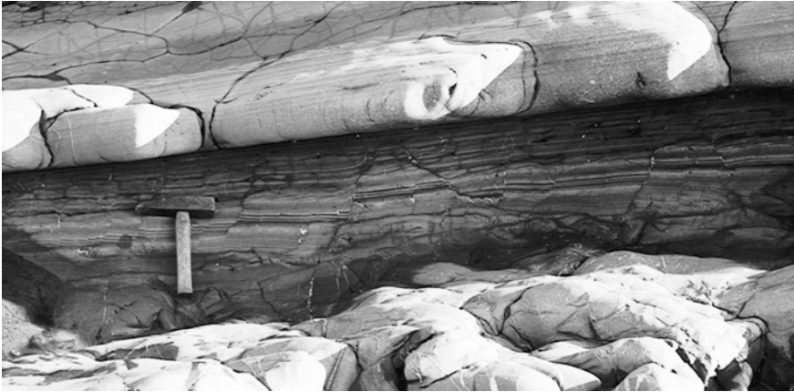
Fig. 3.30 An incompetent shale layer showing extension faults in a chevron fold limb (Bude, England) (after Dubey and Behzadi 1981)
