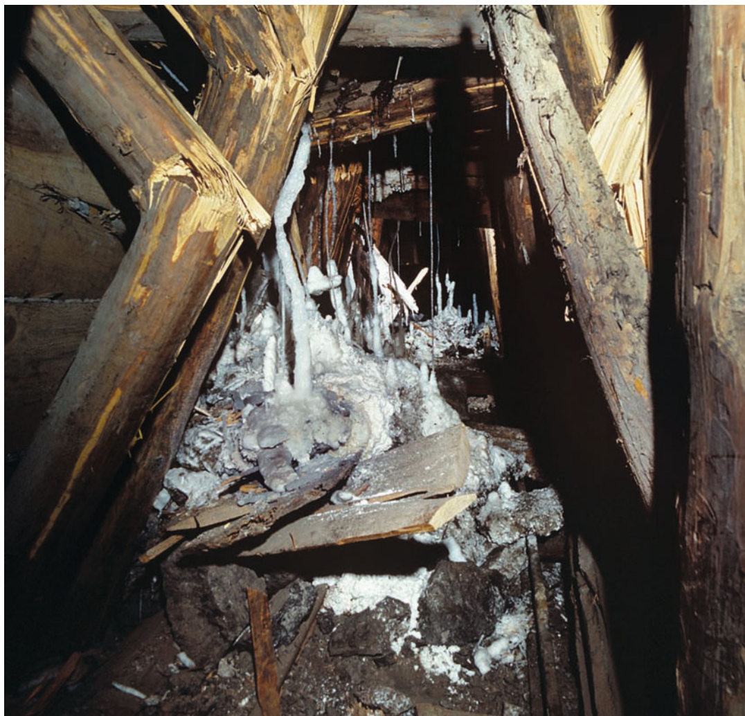
(above) A blind shaft Zergoller with rotting wood and epsomite stalagmites on the IV th level. – Photo: R. Podobnik (on the opposite page) 40 cm tall velvety yellow melanterite stalagmite on the VI th level. Photographed around 1988 – Photo: R. Vidrih
