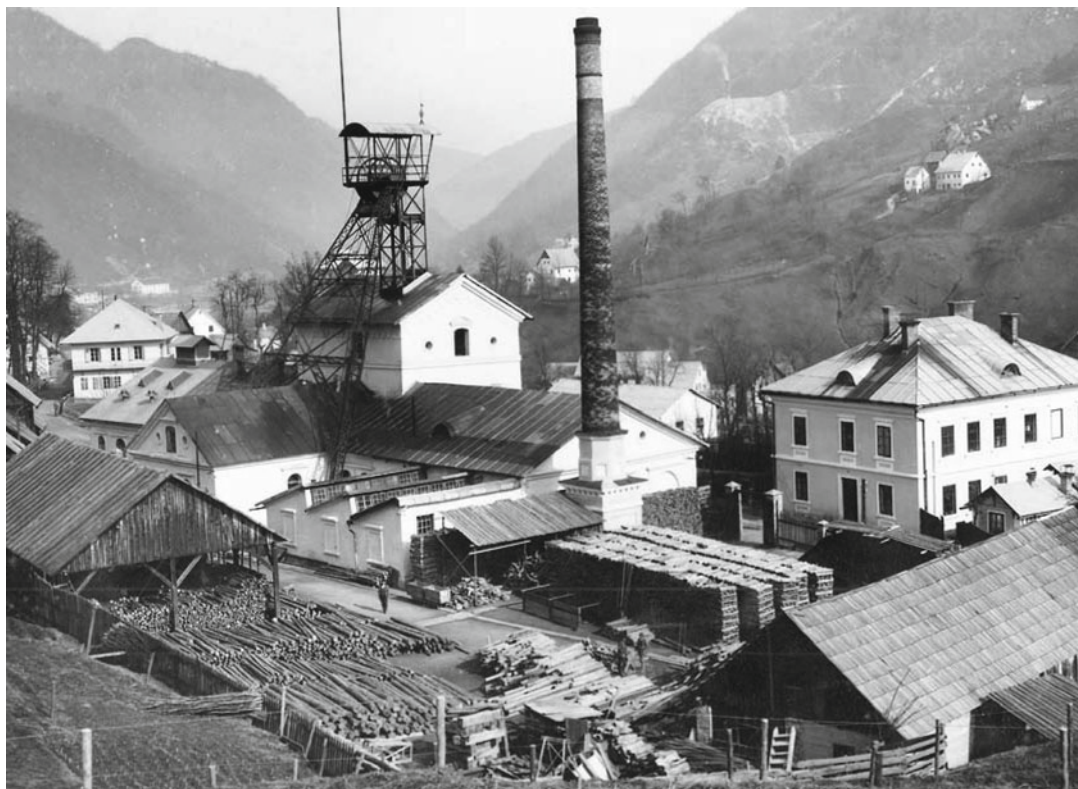
(above) Joseph's shaft with timber storage. After World War II the shaft was renamed as Delo. Here was the main access to the deepest levels of the mine, and also to the mineralogically interesting Grüber Fault zone. Today, the mine is geomechanically stabilized. The water level is presently at the IX th level, and it will gradually rise to the VII th level. (left) An old ore separation (Bašerija) with wagons of ore prepared for smelting around 1900. Photo archive of the Municipal Museum of Idria – Photo: M. Papež
