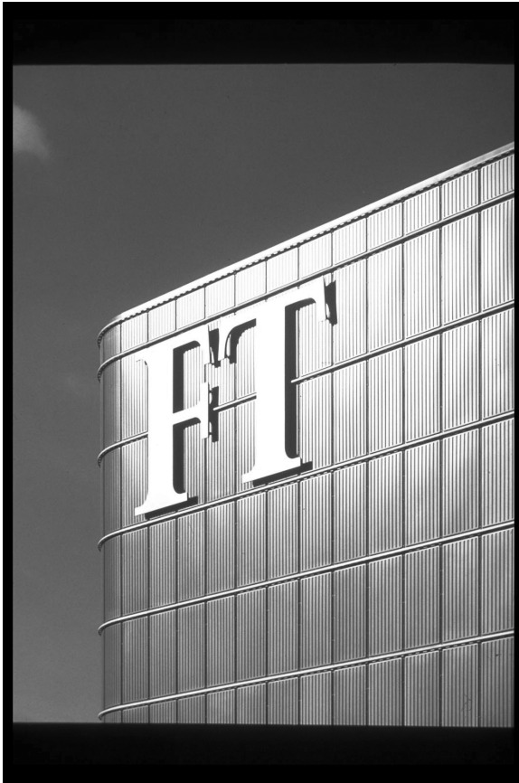
11.4 Architectural application of superplastically formed AA5083 (courtesy Superform Aluminium).
