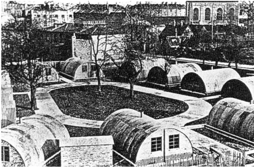
Figure 6.3. A group of emergency Nissen huts built in response to the damage caused by the V2 rocket bombs. (Source: Building , Vol 20, March, 1945)
