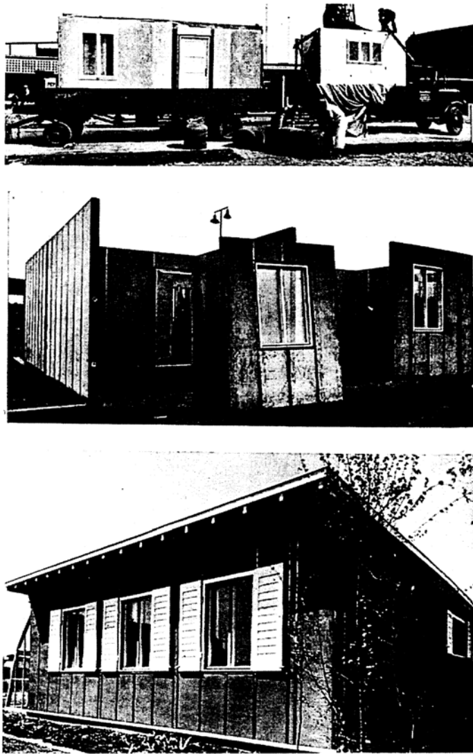
Figure 4.2. Gropius's Copper-Plate houses which were designed for mass production. (Source, Gropius, 1935)
