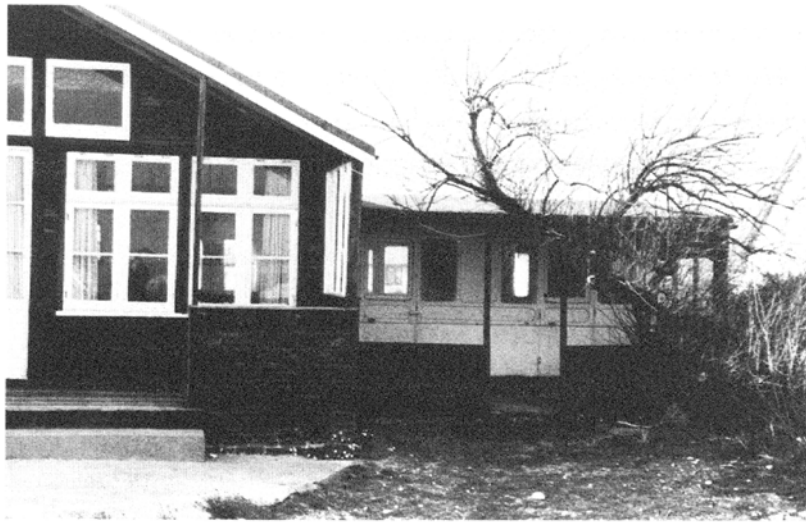
Figure 2.2. Bungalow at Pagham Beach where the original carriage is visible, unaltered externally apart from the addition of a verandah, 1990.
