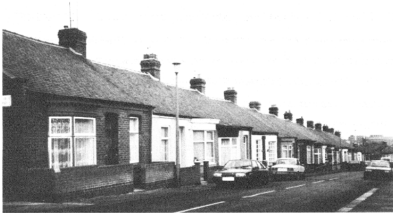
Figure 2.1. Street of single-storey terraced bungalows in Sunderland, 1994.
