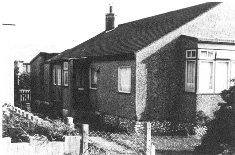
Figure 2.3. Two railway carriages with a pitched roof added across them form this bungalow at Pagham Beach (the tumble-home of the carriage is clearly visible).
