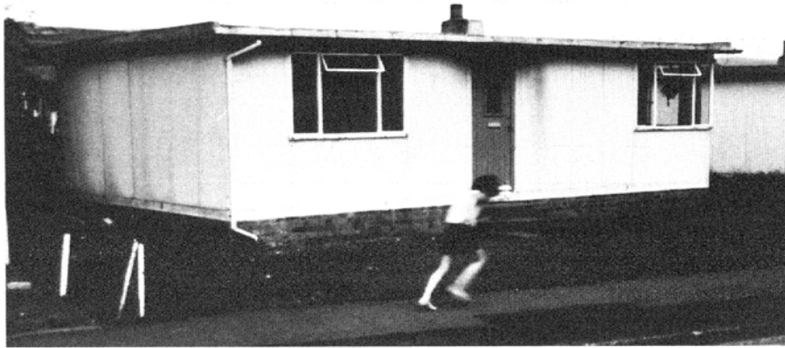
Figure 1.6. Uni-Seco bungalow in Kirkconnel, Scotland, 1986.
