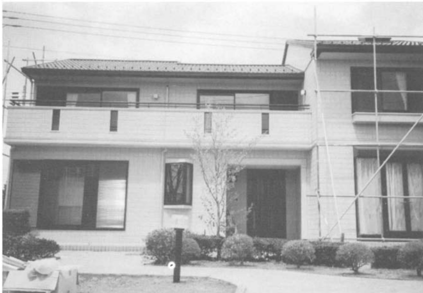
Figure 7.10 Assembled prefabricated building units.
