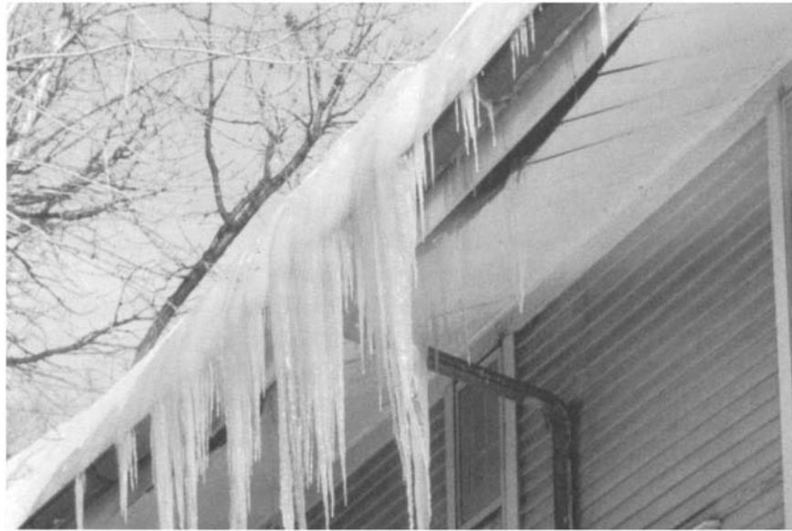
Figure 4.5 Ice dams are common in many cold climate regions.
