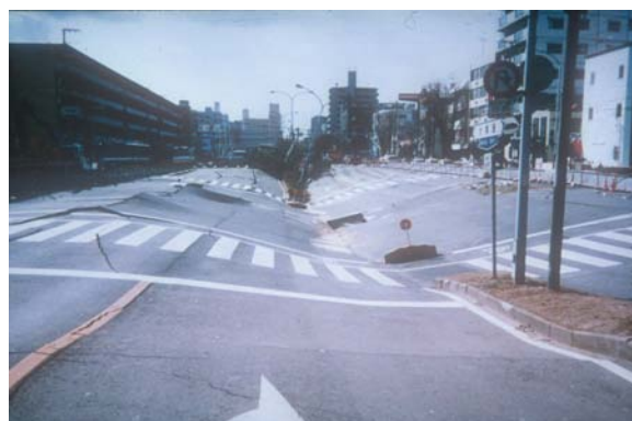
Fig. 13.5 Ground subsidence above Daikai subway station (by Nozomu Yoshida)
