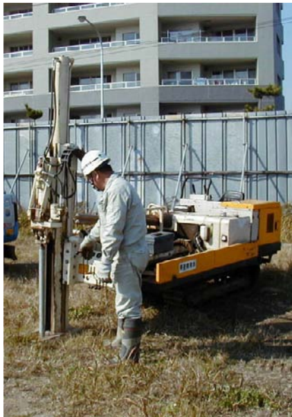
Fig. 26.97 Installation of screen pipe (Zenitaka Corporation)
