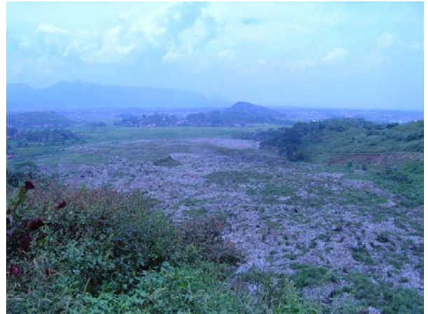
Fig. 10.74 Failure of Leuwigajah landfill near Bandung, Indonesia
