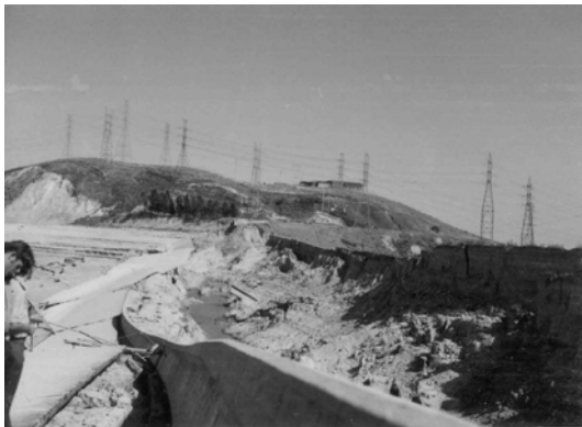
Fig. 17.26 Lower San Fernando Dam after failure (reconnaissance team, Univ. Tokyo)
