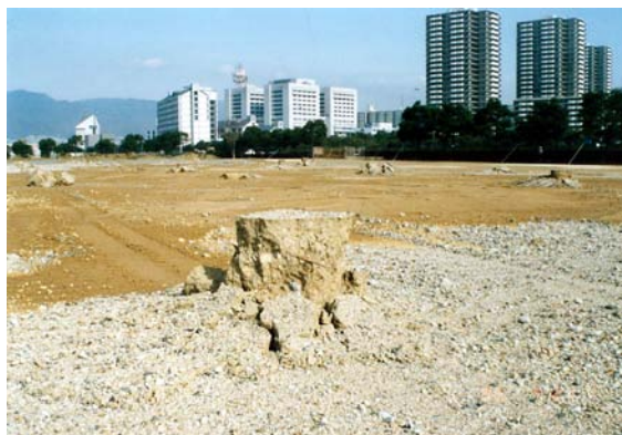
Fig. 17.32 Pile head appearing above subsided ground surface (by K. Ishihara)
