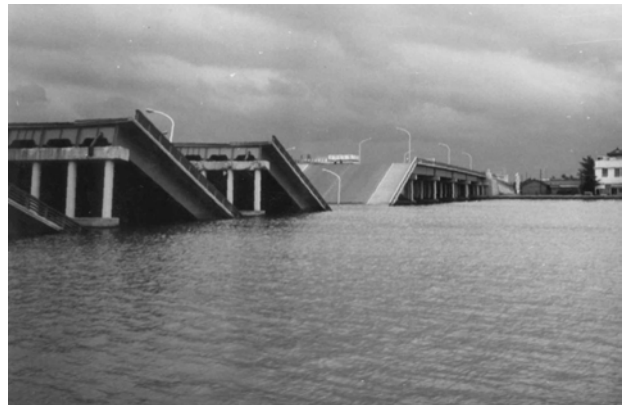
Fig. 24.31 Falling of Showa Bridge in Niigata (Department of Civil Engineering, University of Tokyo)
