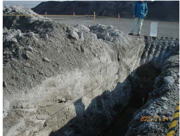
Fig. 10.71 Trench cut in landfill of incinerated ash in Tokyo
