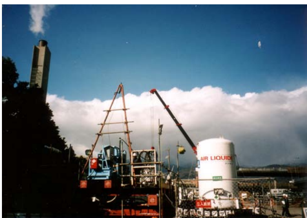
Fig. 10.63 Practice of in-situ freezing (in Uozaki)
