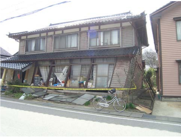
Fig. 5.41 Tilting towards direction of no wall rigidity Fig. 5.42 Dislocation of house from foundation
