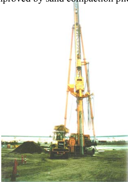
Fig. 26.52 Machine for construction of sand compaction pile
