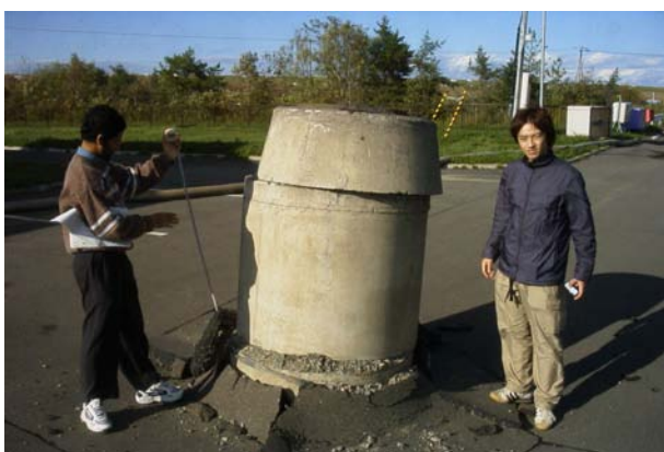
Fig. 17.15 Floating of buried gasoline tank (by Dr. A.A. Acacio)
