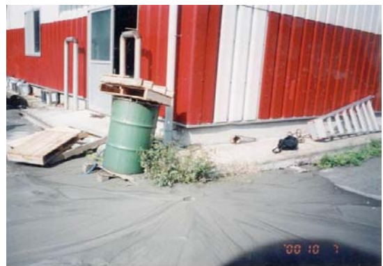
Fig. 17.39 Boiled sand in Takenouchi Industrial Park
