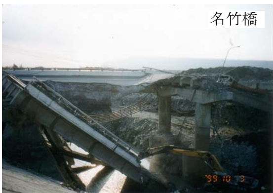
Fig. 14.21 Total collapse of road bridge in Taiwan, 1999 (after 1999 ChiChi earthquake in Taiwan)
