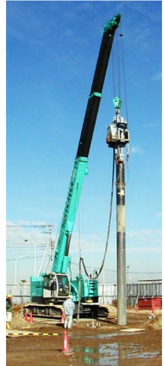
Fig. 26.98 Artificial vibration by pile driver (Zenitaka Corp.)
