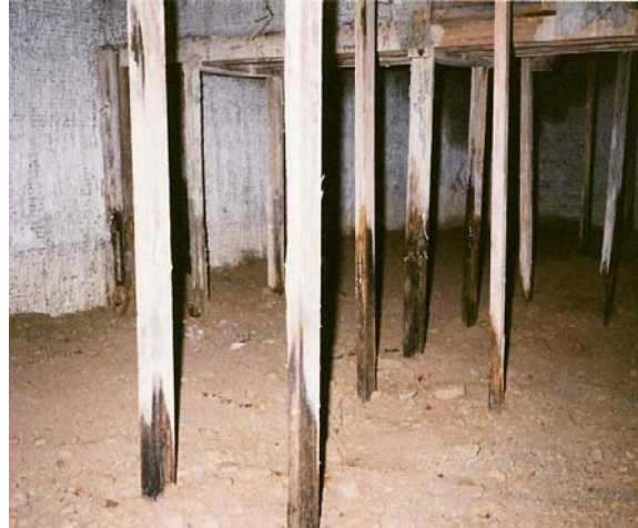
Fig. 26.113 Ground surface without sand boiling after Kobe earthquake inside lattice wall (timber columns are temporary supports during excavation (photograph by Takenaka Corporation))
