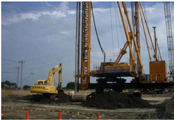
Fig. 26.104 Construction machine for deep mixing method
