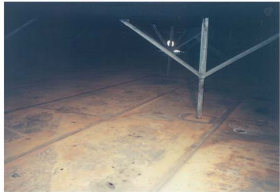
Fig. 26.25 Bottom plate of a storage tank
