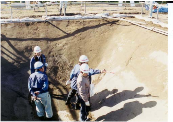
Fig. 18.12 Overall view of excavation at liquefaction site in Sekiyado
