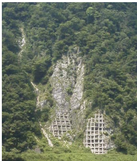
Fig. 26.4 Stabilization of unstable slope by reinforcement
