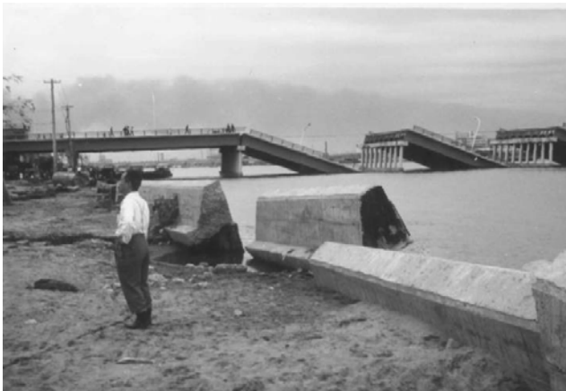
Fig. 17.1 Distortion of quay wall along Shinano River and falling of Showa Bridge in Niigata, 1964 (Department of Civil Engineering, University of Tokyo)
