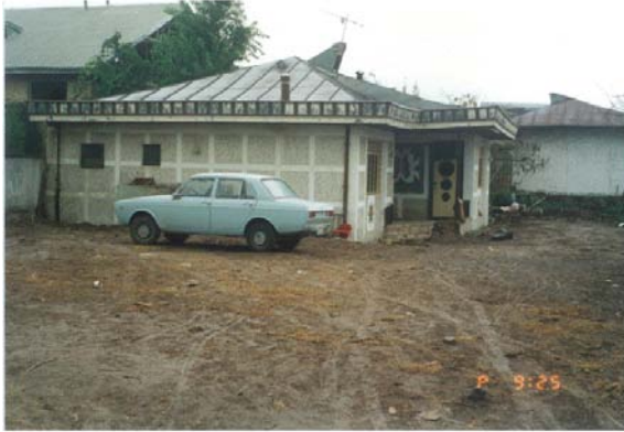
Fig. 17.58 Liquefaction under private house (Gilan, Iran in 1990)
