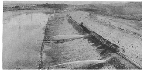
Fig. 17.27 Semi-hydraulic filling for dam construction around 1925 in Taiwan (Furukawa, 1989)
