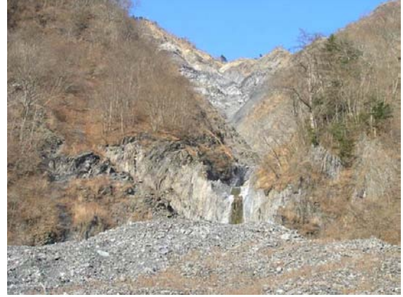
Fig. 15.10 Unstable mountain slope
