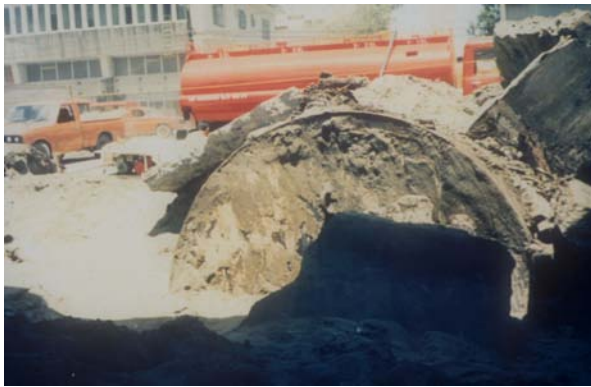
Fig. 17.15 Floating of buried gasoline tank (by Dr. A.A. Acacio)
