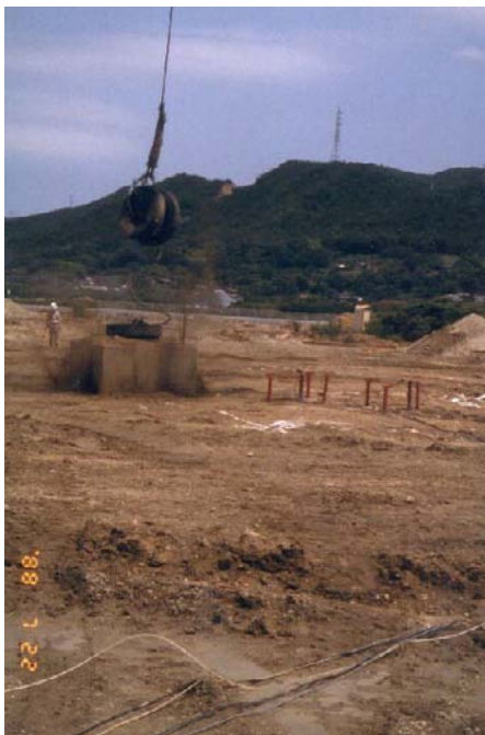
Fig. 26.67 Impact on ground surface made by free fall of weight (at Mizushima)
