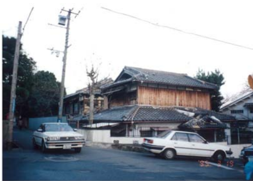
Fig. 5.30 Undamaged wooden house in Kobe (1995)
