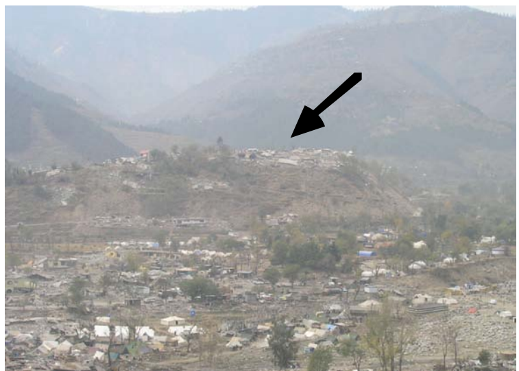
Fig. 6.33 Completely destroyed houses on terrace hill in Balakot of Pakistan during 2005 earthquake
