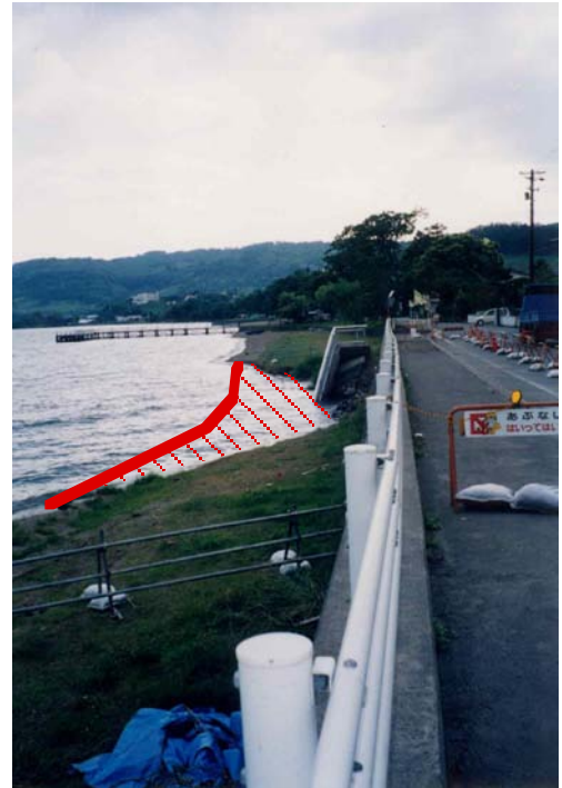
Fig. 15.54 Earthquake-induced failure of caldera wall (Tohya Lake, 1993)
