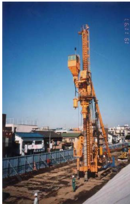
Fig. 26.86 Construction machine for gravel drain
