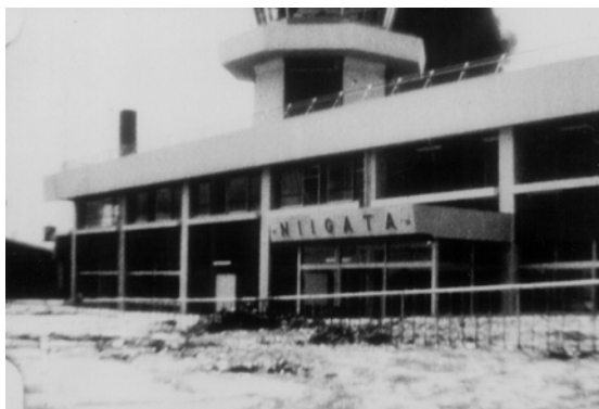
(b) Boiling of sand and water
