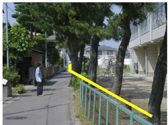
Fig. 25.30 Dislocation of pine trees due to lateral ground displacement in Ohgata, Niigata
