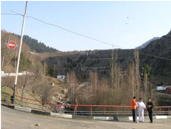
Fig. 26.6 Debris dam near Medeo of Almaty in Kazakhstan (150 m high and 530 m long)
