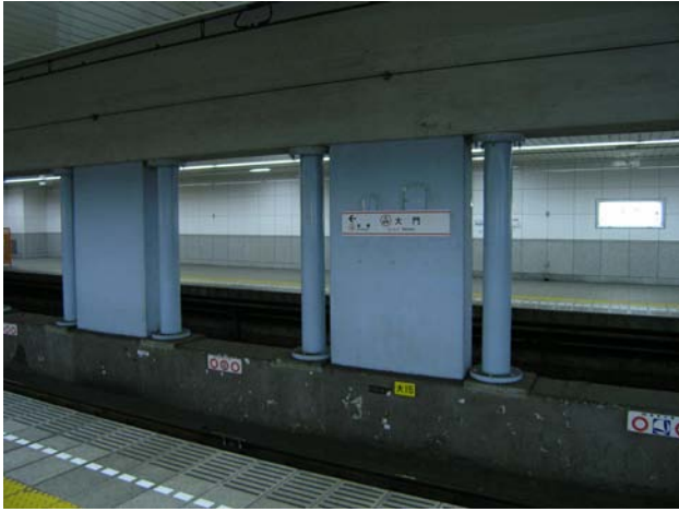
Fig. 13.6 Reinforced central columns in Kasuga Station of Tokyo Metropolitan Subway
