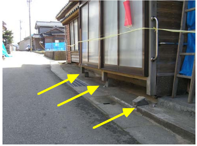
Fig. 5.41 Tilting towards direction of no wall rigidity Fig. 5.42 Dislocation of house from foundation
