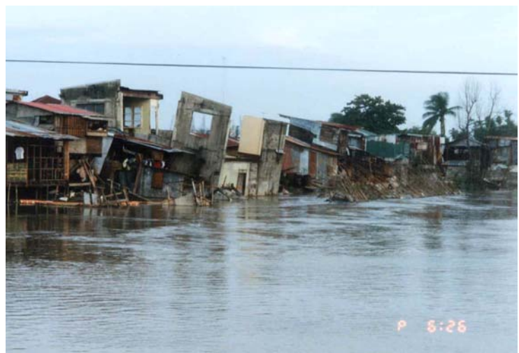
Fig. 17.23 Lateral movement of embankment in Dagupan
