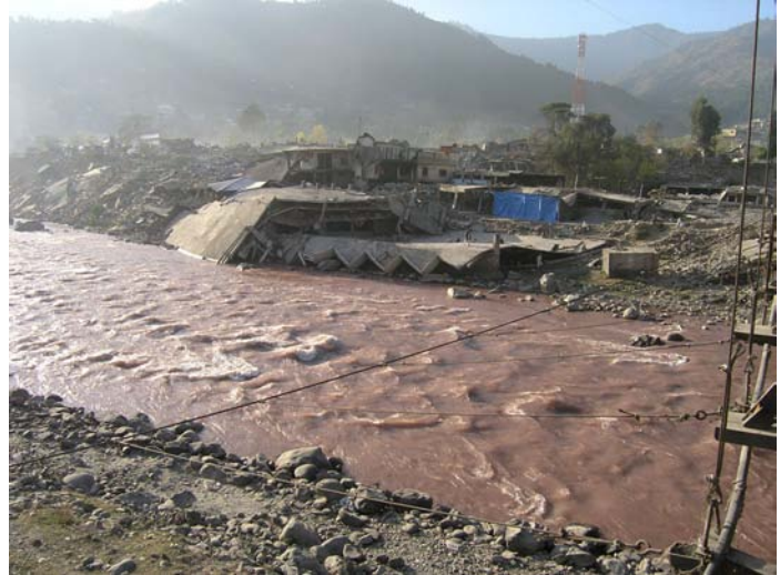
Fig. 5.40 Total collapse of buildings in Balakot, Pakistan, in 2005
