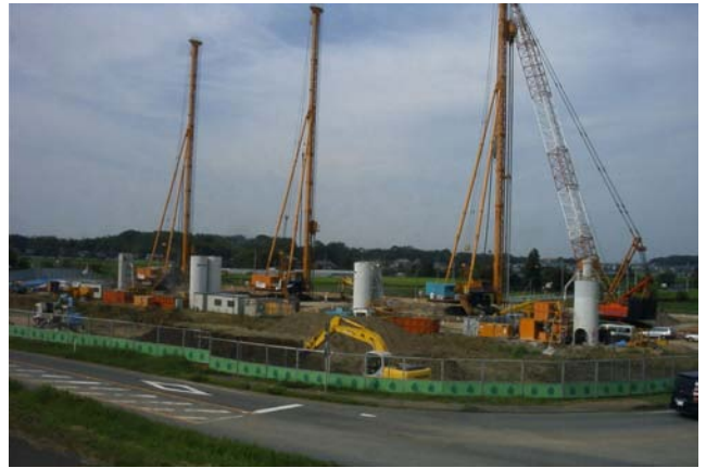
Fig. 26.103 Deep mixing of liquefiable sand for reinforcement of river dike
