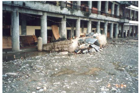
Fig. 17.16 Floating of sewage tank
