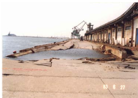
Fig. 24.8 Substantial damage of sheet-pile wall at Akita Harbor in 1983 (by Dr. K. Wakamatsu)
