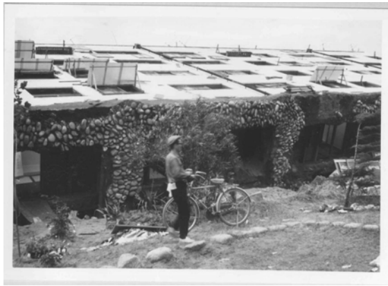
Fig. 17.7 Base of Kawagishi-cho apartment building after falling (Department of Civil Engineering, University of Tokyo)
