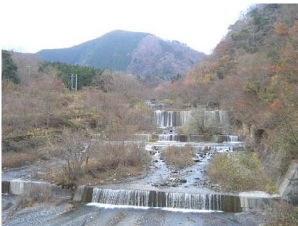
Fig. 15.12 Erosion control dams in Abe river channel
