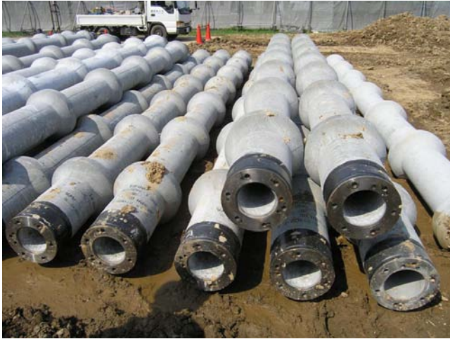
Fig. 13.31 Nodular piles prior to installation
