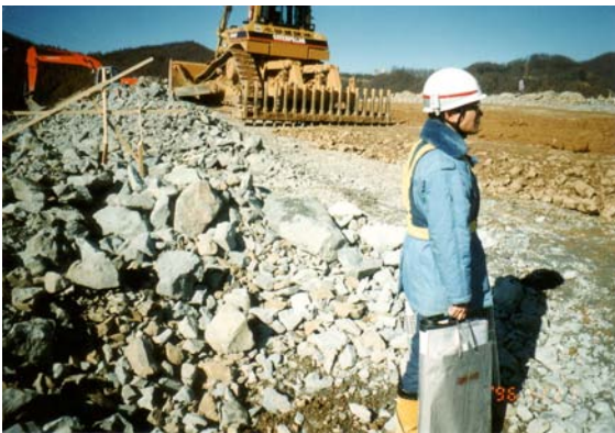
Fig. 10.51 Construction of rock fill dam
