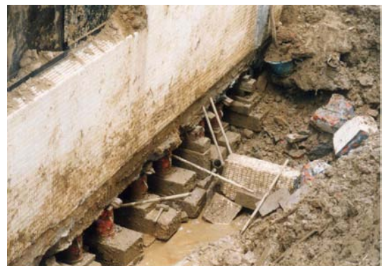
Fig. 17.65 Ongoing jacking up of house foundation (in Taiwan)
