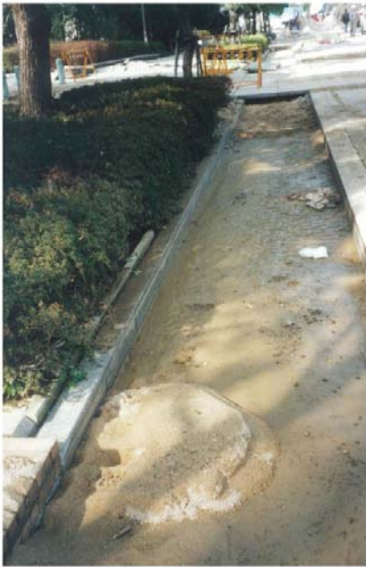
Fig. 18.44 Minor liquefaction in Higashi Park on inland side of original coast line in Kobe
