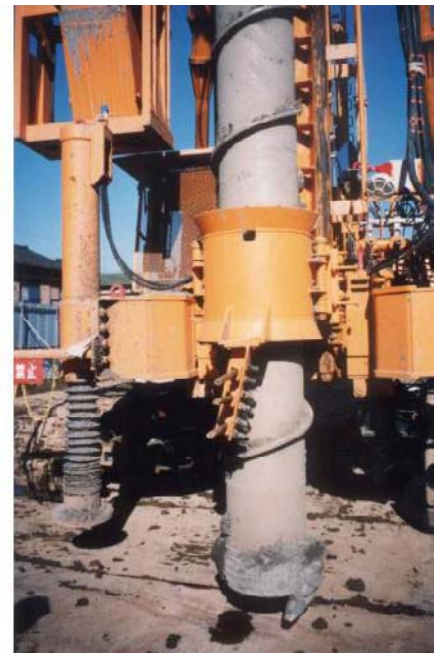
Fig. 26.86 Construction machine for gravel drain
