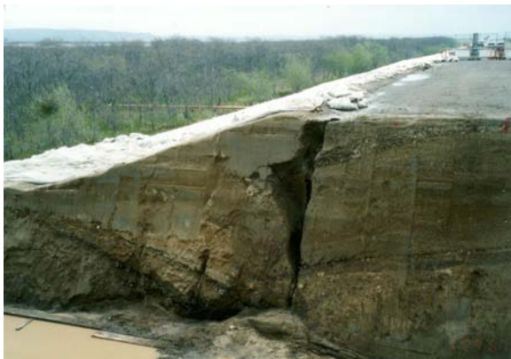
Fig. 17.10 Excavation of damaged Tokachi-river dike
