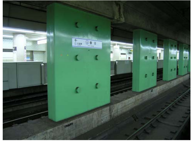
Fig. 13.7 Reinforced central columns in Daimon Station of Tokyo Metropolitan Subway
