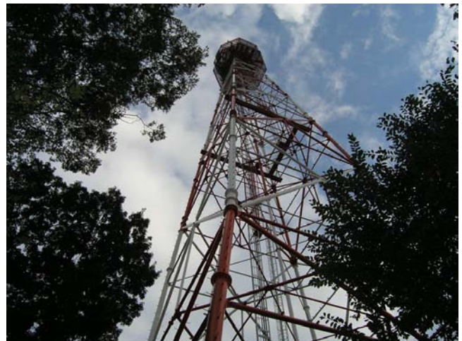
Fig. 23.18 Data transmission tower in Kodaira, Tokyo
