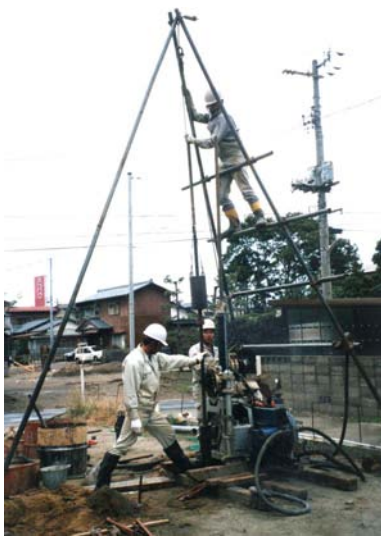
Fig. 8.10 Practice of standard penetration test
