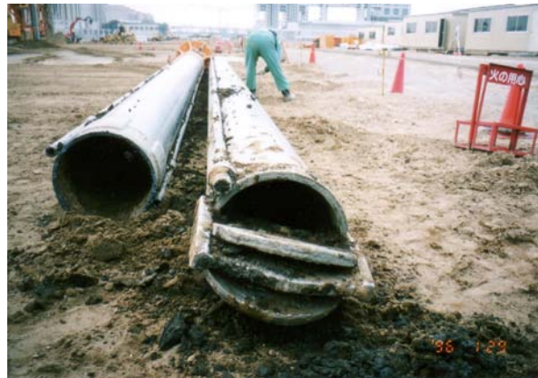
Fig. 26.53 Bottom of casing
