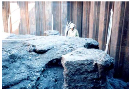
Fig. 26.117 Excavation of soil mass solidified by silica grouting
