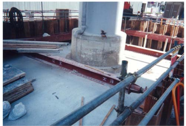
Fig. 24.66 Increasing lateral resistance of pile foundation by enlargement of pile cap and increasing number of piles (in the center of Sunnomiya, Kobe)
