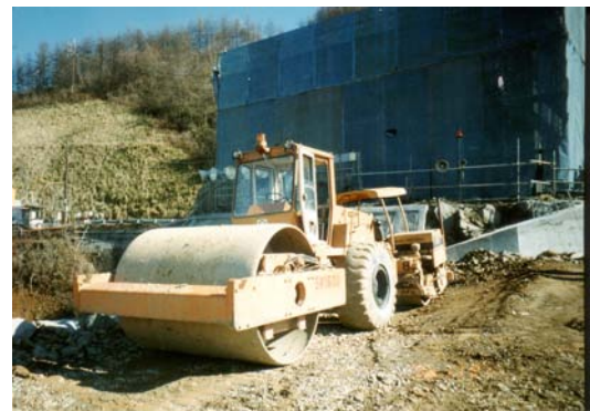
Fig. 17.29 Soil compaction for dam construction
