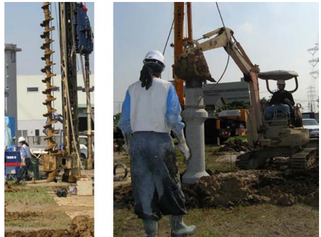
Fig. 13.32 Installation of nodular pile
