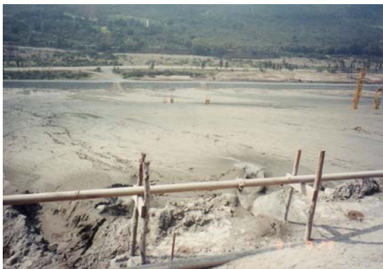
Fig. 20.22 Discharging coarse material onto downstream slope of tailing dam (Lomeral in Chile)
