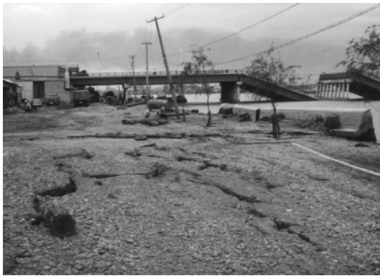
Fig. 17.20 Sheet pile wall near Showa Bridge in Niigata, 1964 (Dept. Civil Engineering, University of Tokyo)
