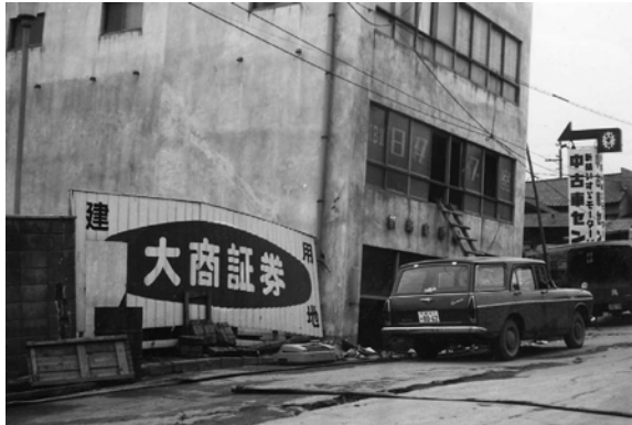
Fig. 17.50 Subsidence of building in liquefied area in Niigata, 1964 (Department of Civil Engineering, University of Tokyo)
