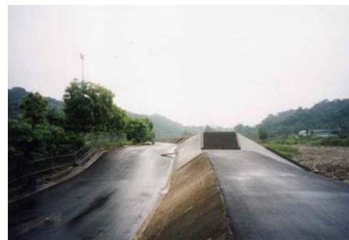
Fig. 14.3 Repaired shape of dike in Wufeng
