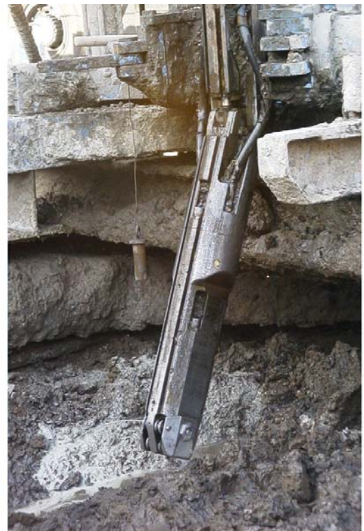
Fig. 27.8 Soil improvement of peaty material by grouting special liquid
