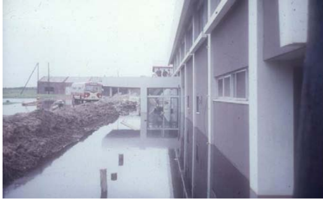
Fig. 25.57 Terminal building of Niigata Airport after liquefaction and subsidence (Department of Civil Engineering, University of Tokyo)
