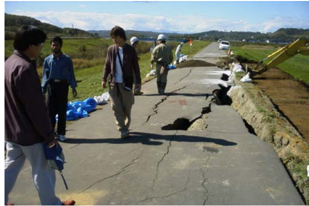
Fig. 17.14 Quick restoration after 2003 Tokachi earthquake
