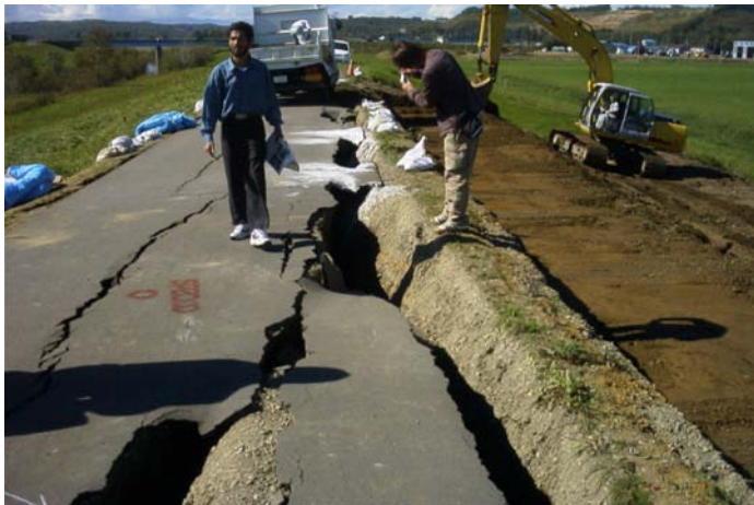
Fig. 14.23 Quick restoration in dike of Ushishubetsu River in Hokkaido
