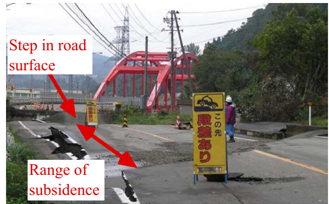
Fig. 14.16 Bridge out of service due to subsidence of approach embankment (Minami Yamabe Bridge of Ojiya City, 2004 Niigata-Chuetsu earthquake)
