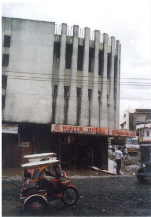
Fig. 17.56 Subsidence and tilting of building in Dagupan, Luzon, in 1990
