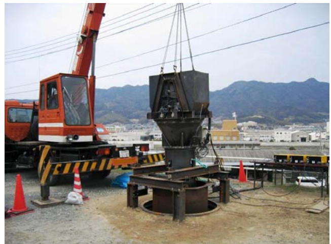
Fig. 26.61 Machine for insitu ultrasonic compaction of sand (Oh-uchi and Murakami, 2006)
