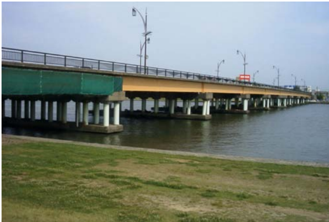
Fig. 24.65 Present foundation of Showa Bridge after reconstruction
