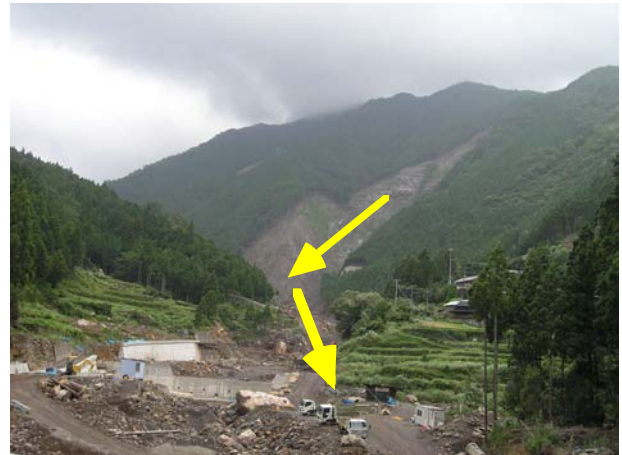
Fig. 15.60 Changed flow direction of debris at bottom of slope (rainfall-induced slope failure in Shikoku, Japan, in 2004)
