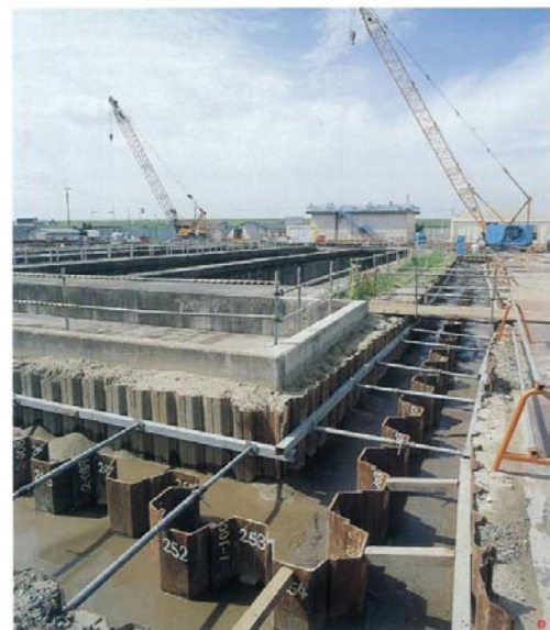
Fig. 26.92 Appearance of sheet pile wall with drains (Sumitomo Metal Industries)
