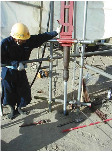
Fig. 26.97 Installation of screen pipe (Zenitaka Corporation)
