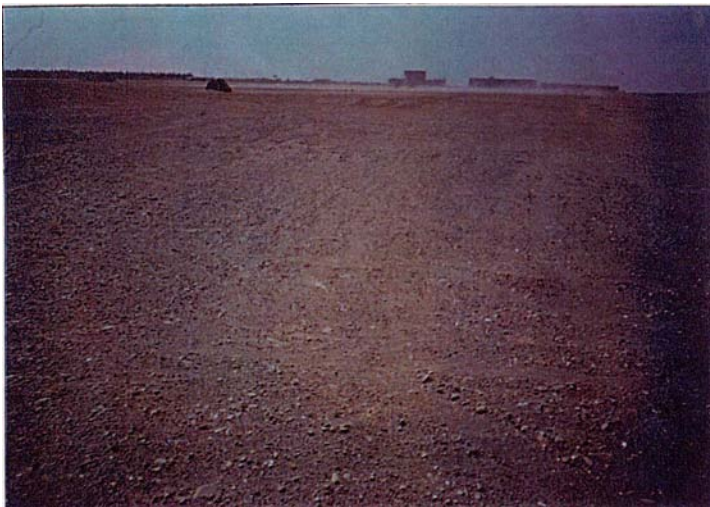
Fig. 26.71 Satisfactory effects of sand densification by dynamic consolidation in Lu-kang, Taiwan (Kaiyo Kogyo Company)
