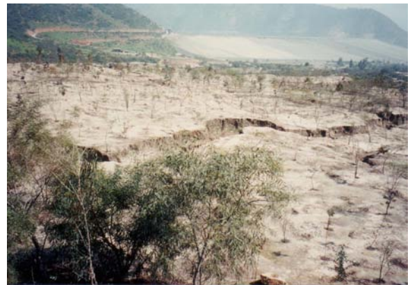
Fig. 20.21 Site of tailing dam failure in El Cobre, Chile
