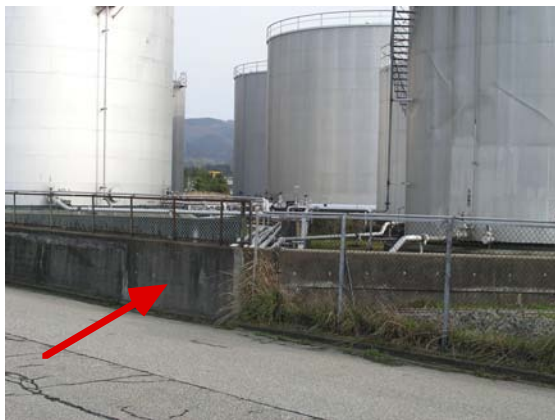
Fig. 26.26 Wall surrounding storage tanks (in Nanao Harbor)
