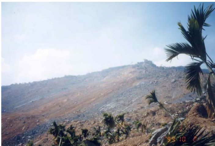
Fig. 15.37 View of Jiu-Feng-Er-Shan landslide
