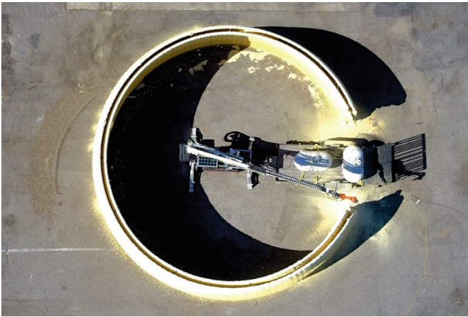
Fig. 2. Digital construction platform ( http://matter.media.mit.edu/ ).
