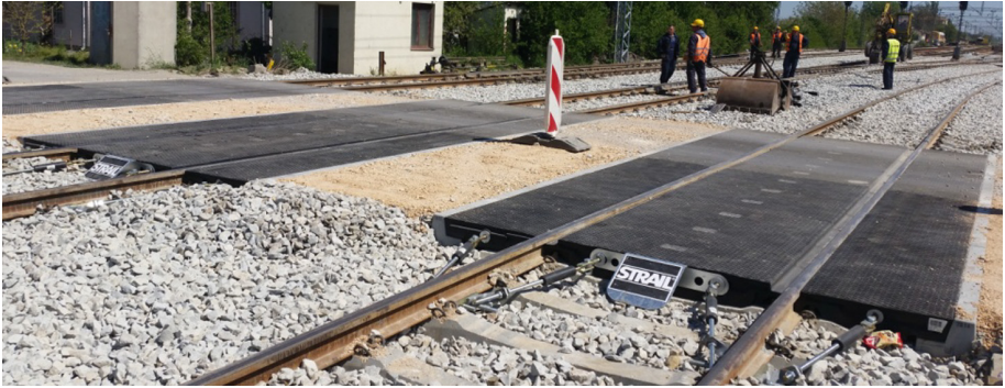
Fig. 12. Installation of rubber panels on railway line Belgrade - Pančevo in 2015.
