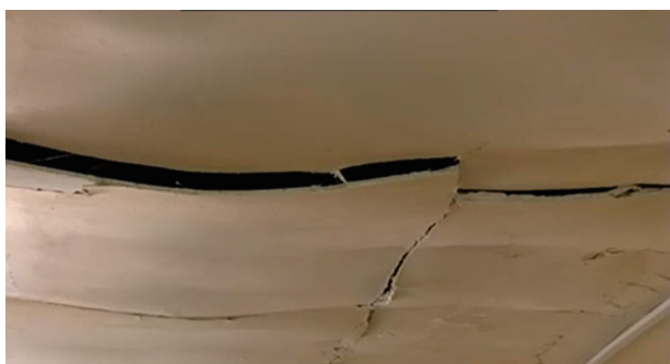
Fig. 10. Cracked ceiling.
