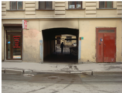
Fig. 3. Vehicular passage to the courtyard.
