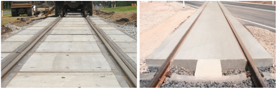
Fig. 13. Reinforced concrete slabs made of precast concrete [4, 6].
