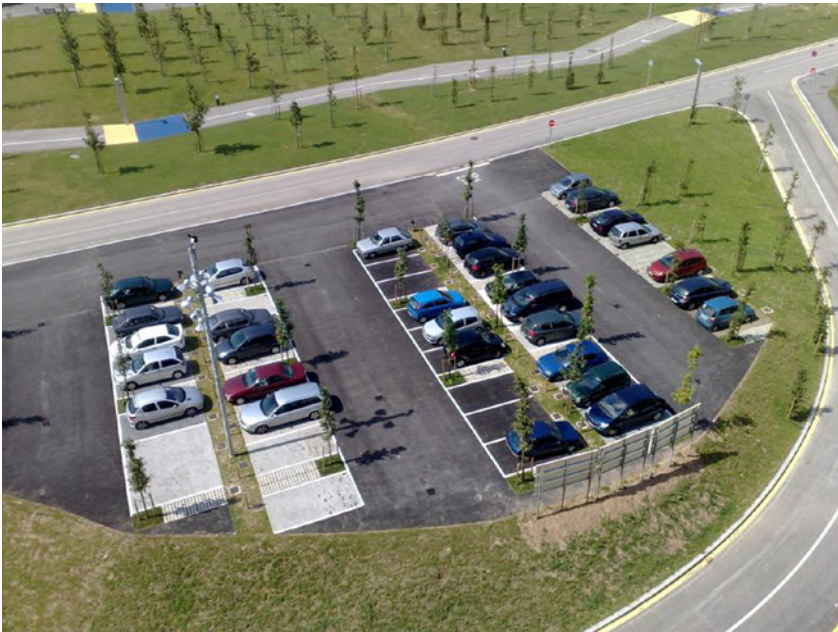
Figure 23.3 PPS car park of various designs constructed for the purpose of long-term monitoring, Santander (Spain).
