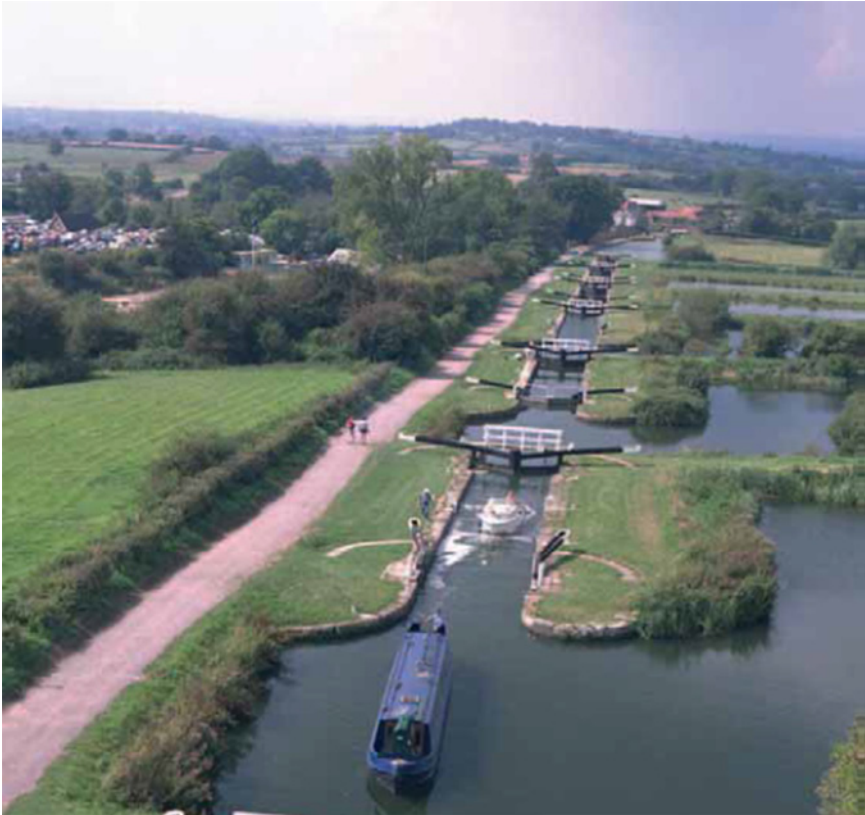
Figure 14.1 Water storage area (to the right) situated next to each lock chamber (black and white gated structures on left) at the Caen Hill flight, Devizes (UK). Copyright Chris Talbot and licensed for reuse under the Creative Commons Licence.
