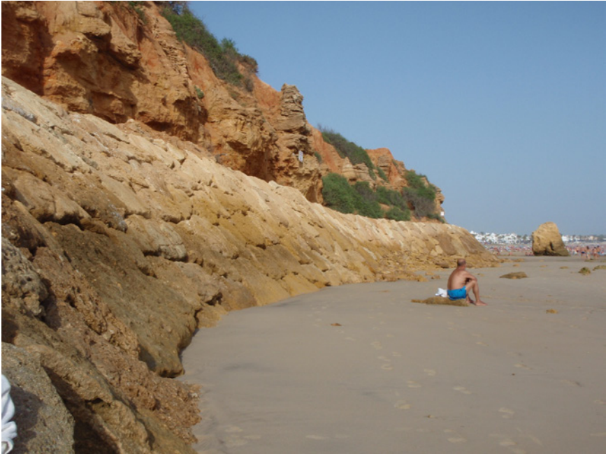
Figure 18.2 Defensive sea wall, near Cadiz (Spain).
