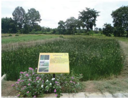
Figure 25.2 Examples of constructed wetlands for wastewater management: (a) combined pond and wetland system for treatment of urban stormwater, Edmonton (Canada); (b) horizontal subsurface flow wetland with two parallel treatment lines treating gully pot effluent, Fife (Scotland); (c) surface flow wetland planted with sedge grass ( Cyperus tegetiformis ) treating wastewater from a brewery near Khon Kaen (Thailand). The treated water is recycled for irrigation of a golf course (photo reproduced by permission of Dr Netnapid Tantemsapya, Khon Kaen University, Thailand); (d) mature constructed wetland, an integral part of an ecological treatment system for managing distillery wastewater, Scotland, and designed by Living Water (photo reproduced by permission of Jane Shields, Living Water Ecosystems Ltd).
