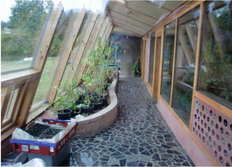
Figure 13.4 Greywater harvesting system planters in Earthship's conservatory.
