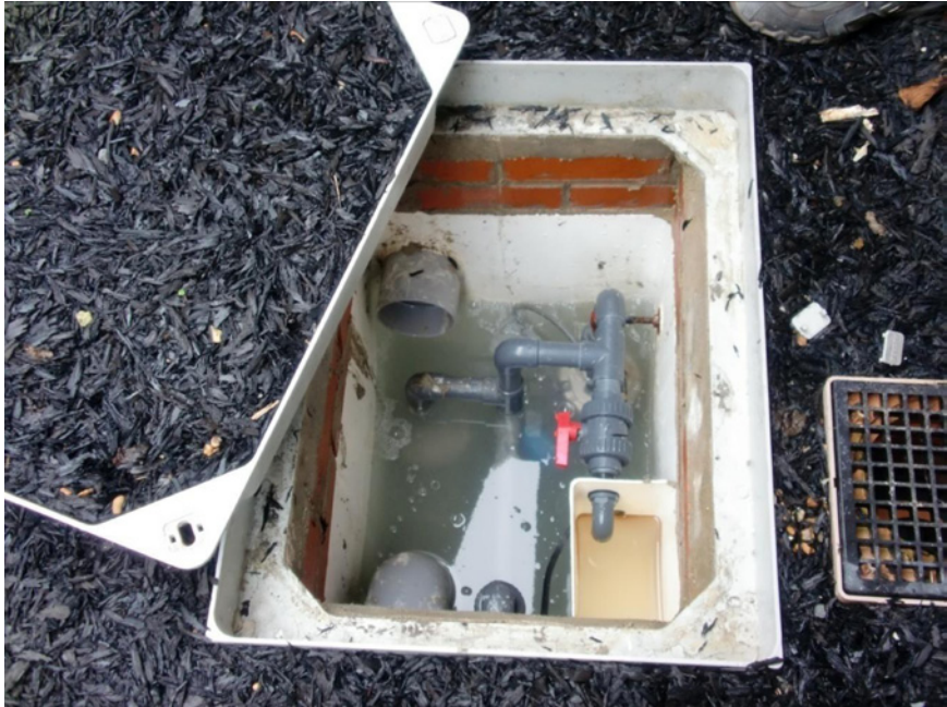
Figure 13.2 Plan view of the exterior greywater tank at the bungalow at Whichelo Place , Brighton.
