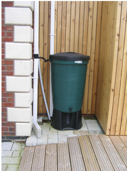
Figure 12.1 An inexpensive domestic rainwater harvesting butt or barrel.
