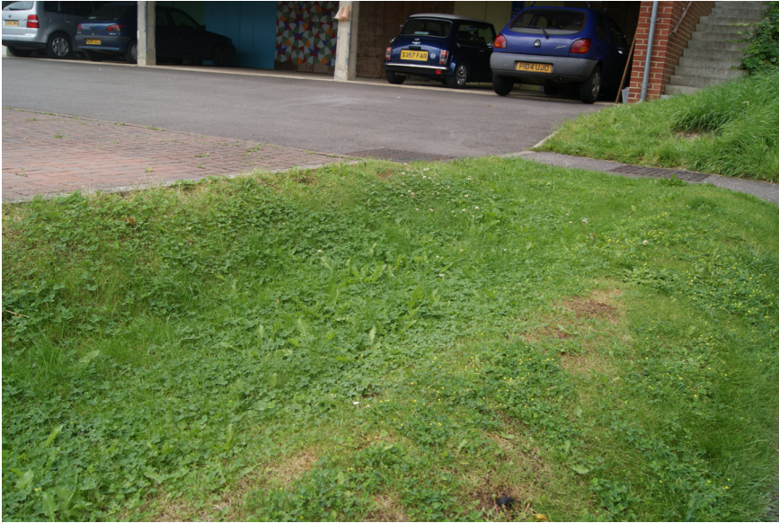
Figure 22.15 Springhill overflow swale.
