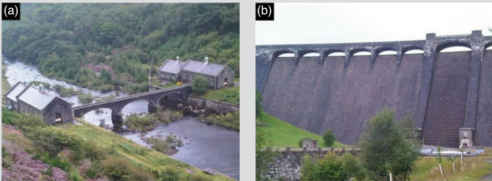
Figure 6.5 Elan Valley turbine houses at (a) Caban Coch (North and South) and (b) Claerwen Dam, where the turbines are housed under the floor level roof in the bottom right-hand corner (taken in 2011).
