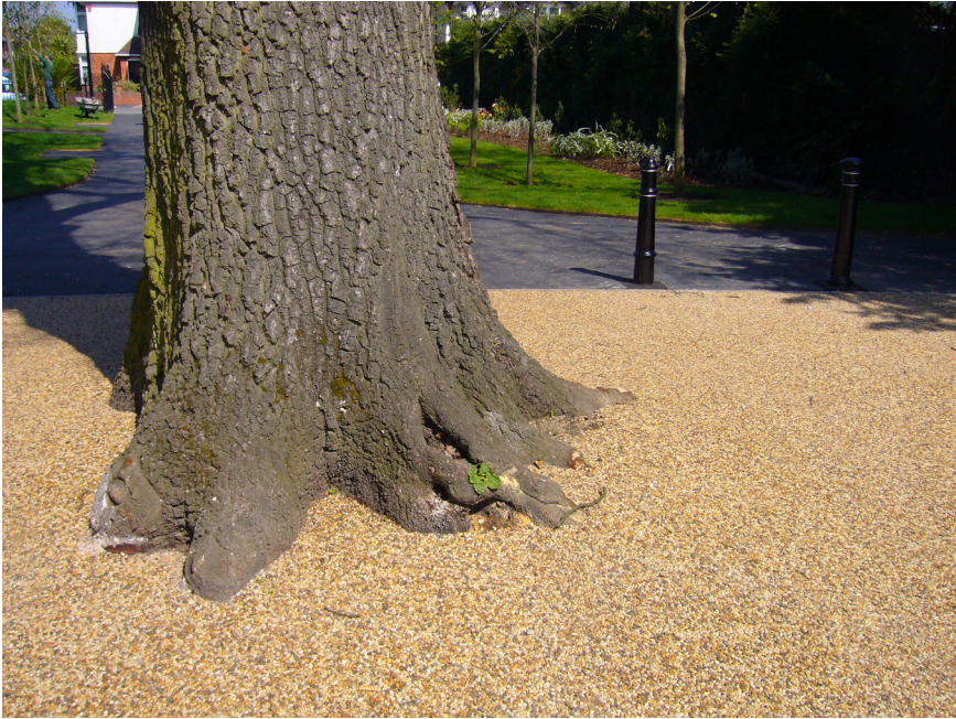
Figure 22.5 Porous resin-bound surfacing, Rugby.
