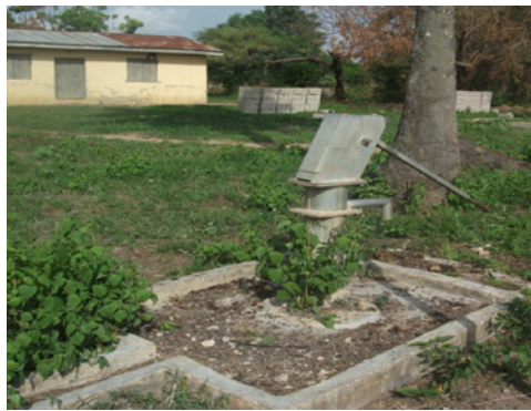
Figure 27.4 A typical picture of an abandoned hand pump borehole constructed between 2005 and 2010 in Mopa Kogi state (Nigeria).
