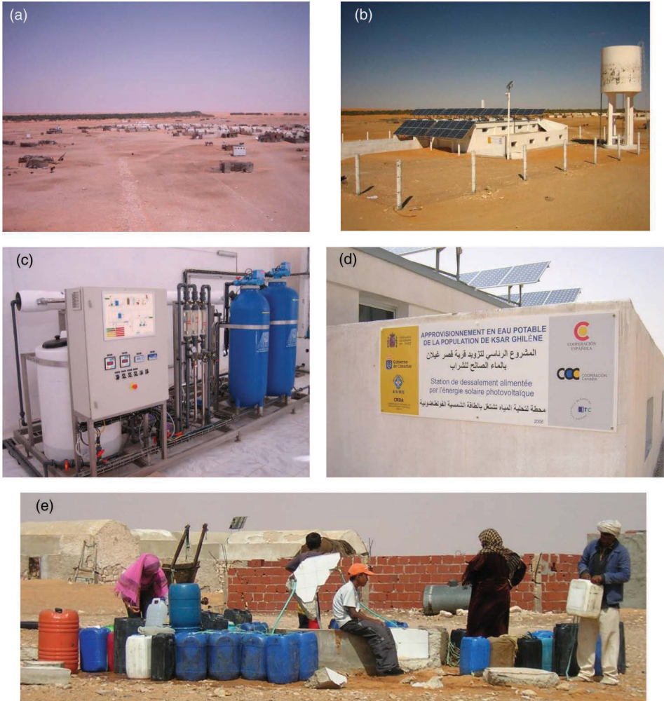
Figure 2.18. Ksar Ghilène plant: (a) situation of Ksar Ghilène; (b) standalone PV-RO plant; (c) brackish water RO plant; (d) funding notice at the Ksar Ghilène plant; (e) one of the five freshwater supply points provided by the plant.
