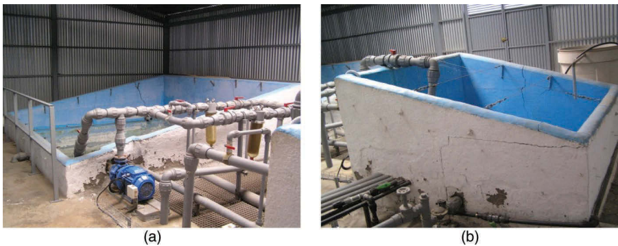
Figure 2.5. (a) PL-2 pool for the feed water to the plant; (b) PL-1 pool for the rejected streams from the plant.
