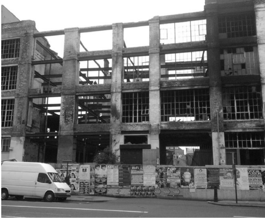
Figure 7. Abandoned building, Commercial Road, London, May 2006.
