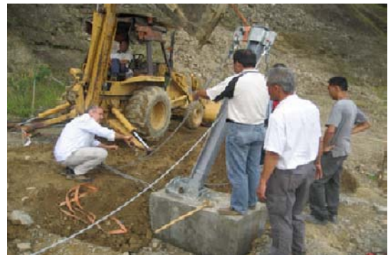
Photo 3 Installation of the Posts in Progress
