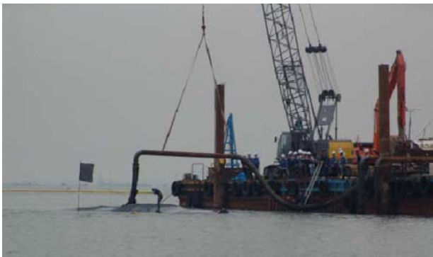
Fig. 11 Equipment combination for tube fillings
