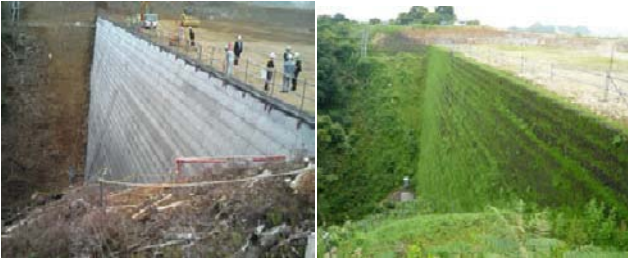
Immediately after completion One year after completion
