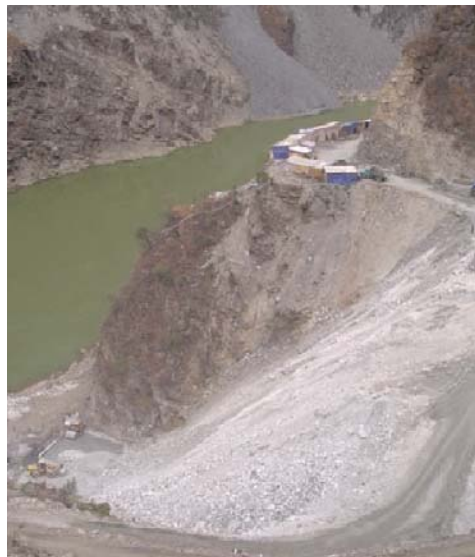
Fig. 1 Start of Construction
