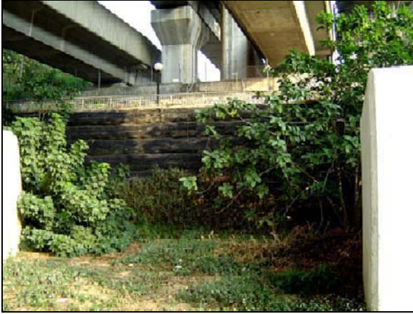
Picture 7 Reinforced fill slope eight years after completion
