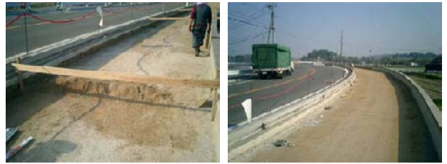
Fig. 5 Digging and leveling
