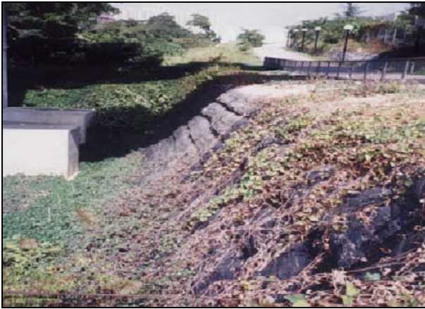
Picture 6 Access road with reinforced fill slope
