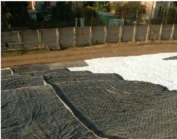
Fig. 6 Laying down of the drainage geocomposite (white) on the GCL (black )
