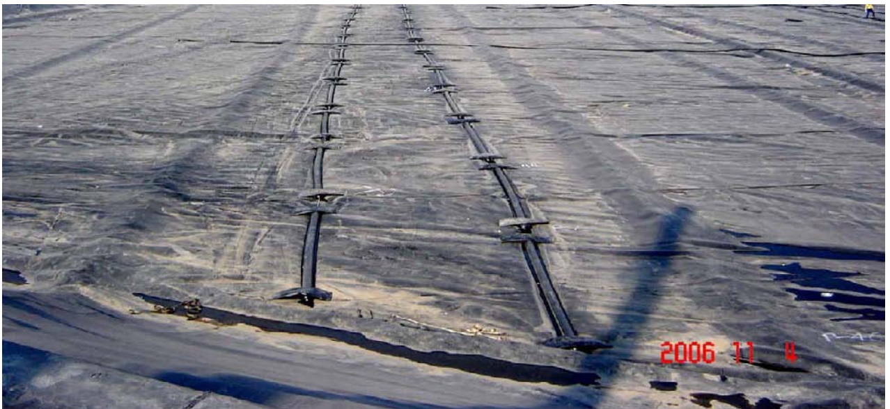
Fig. 5 Matched ballast and floats
