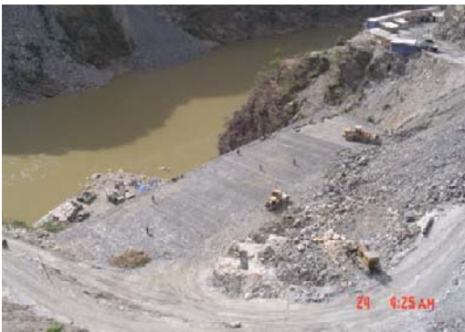
Fig. 2 Construction of geogrid-reinforced slope
