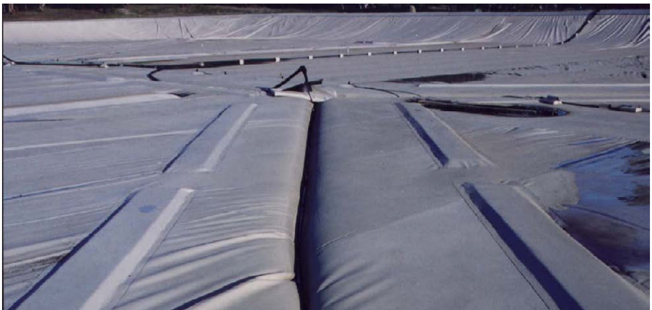
Fig. 1 A floating cover with tension from ballast and floats
