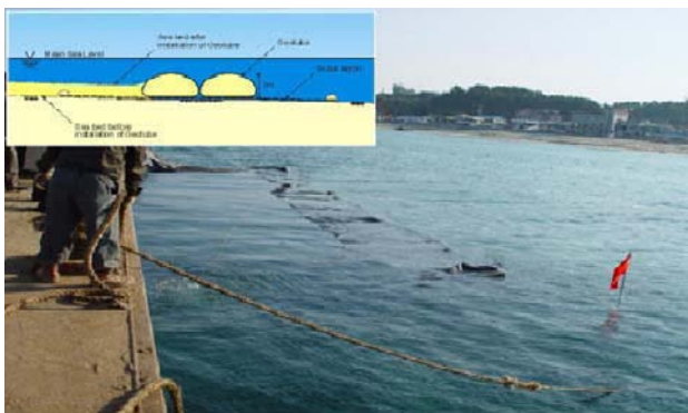
Fig. 1 Geotextile tube breakwater at Yeongjin Port
