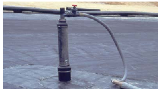
Fig. 1 Connection between geomembrane and gas venting well
