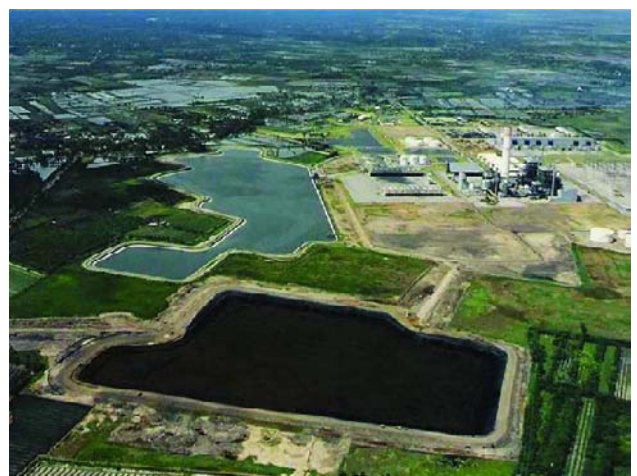
Fig. 3 Overview of the Installed HDPE Lined Ponds
