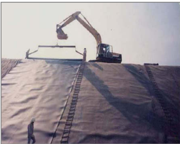
Fig. 4 Deployment of geomembrane in progress
