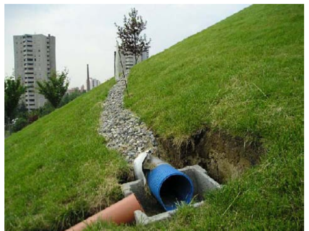
Fig. 9 Intermediate transversal draining trench
