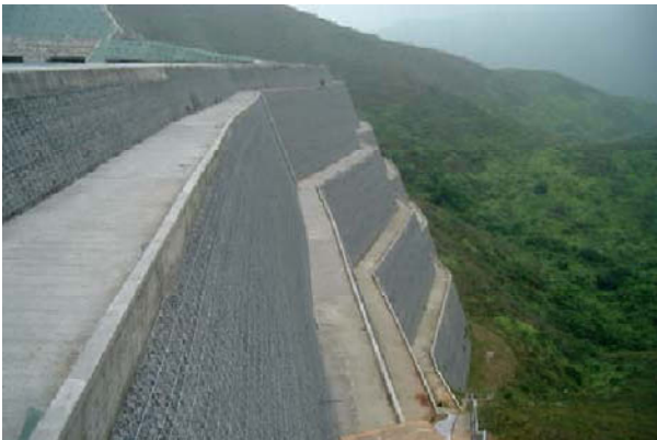
Fig. 5 Completed reinforced fill embankment on the side facing the waste
