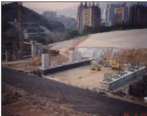
Picture 2 Kwai Chung Park Viaduct overview
