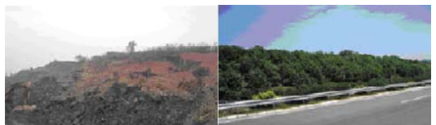
Photo 6 Comparison of untreated treated cut slope from K136+040 to K136+450
