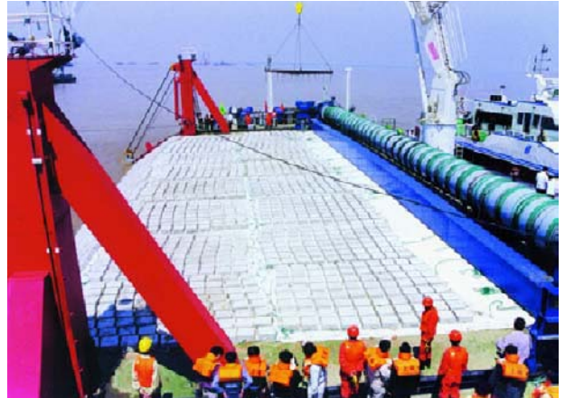
Fig. 4 Large scale mattress laying vessel
