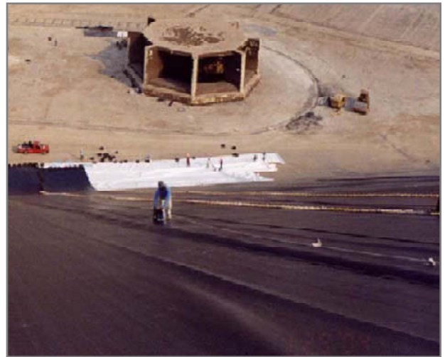
Fig. 5 Welding of geomembrane at project site
