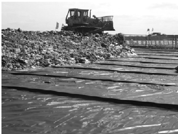
Fig. 7 Placement of solid waste directly over leachate filter geotextile for the Laogang Municipal Solid Waste Landfill Project Phase 4
