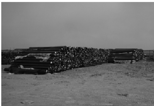
Fig. 8 Stockpile of leachate filter geotextile for the Laogang Municipal Solid Waste Landfill Project Phase 4
