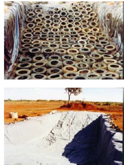
(b) View of cell construction before and after the geotextile installation
