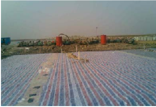
Fig. 4 Pre-compression and vacuum draw
