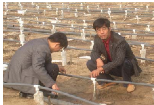
Fig.3 Vacuum system installation
