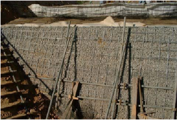
Fig. 3 Completed gravel facing
