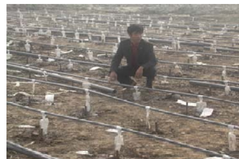
Fig.2 Vacuum system installation
