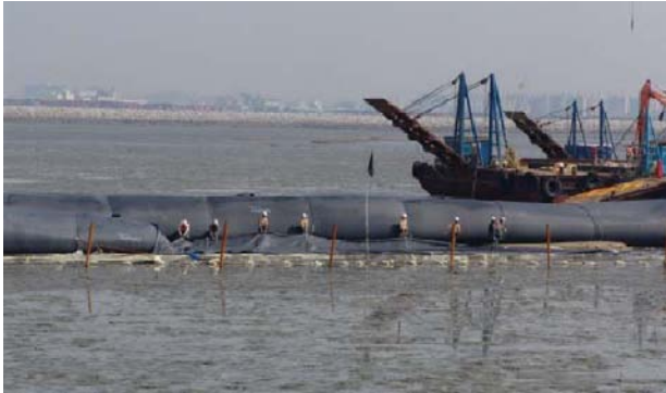
Fig. 10 Geotextile tube deployments using post piles
