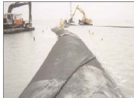
Fig.1 Orbicular shape of geotube
