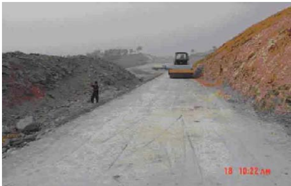
Photo 4 Compaction of fill
