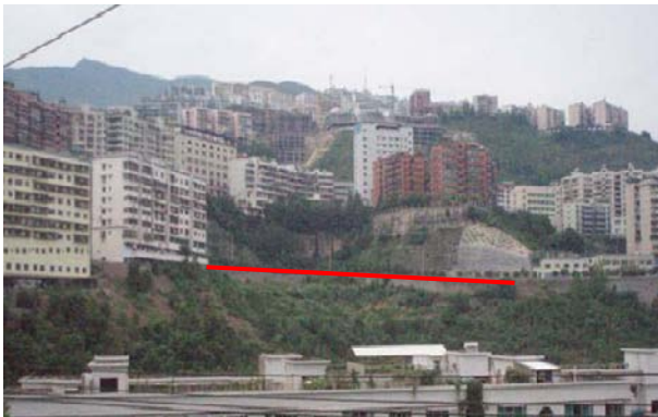
Fig. 1 The photo of the site (the red line shows the new road and the old one was just behind the line)
