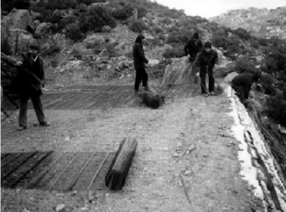
Fig. 1 Continuing lines of geogrid rolls in the field
