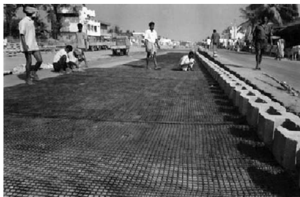
Fig. 3 Geogrid reinforcement and fascia units for NH5, Dharmavaram-Tuni Package
