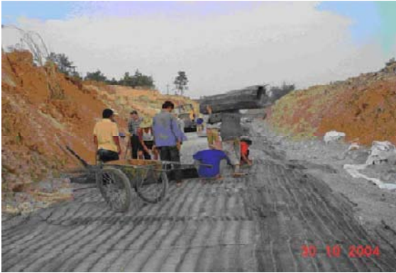
Photo 2 Counter-wrap and pave geogrid
