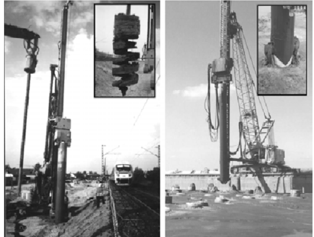
Fig. 2 Excavation and substitution technique with double flap pipe (pictures: Möbius AG)
