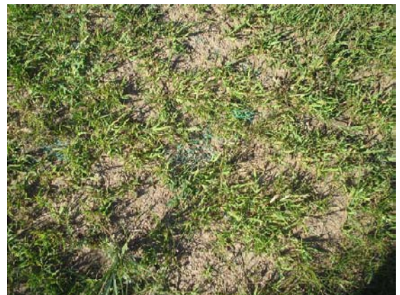
Fig. 5 The effect picture of 3D geonet grass ecological slope protection
