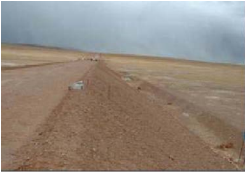
Photo 1 Slope Protection with Geocell
