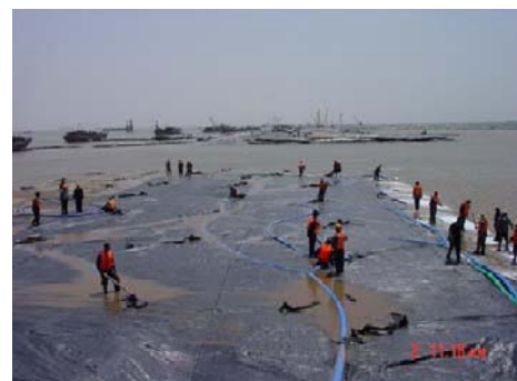
Fig. 2 Flat shape of geotube
