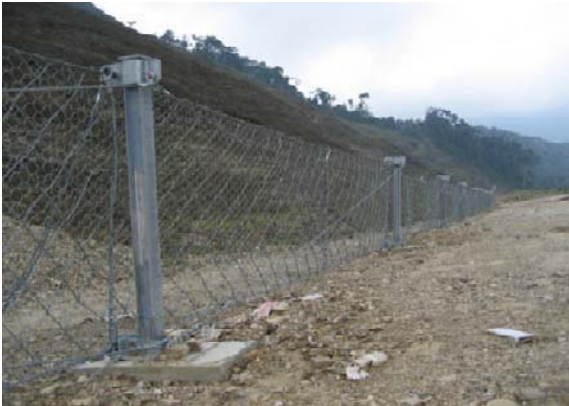
Photo 6 Installed barrier on the upper berm
