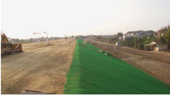
Fig. 4 The trial embankment
