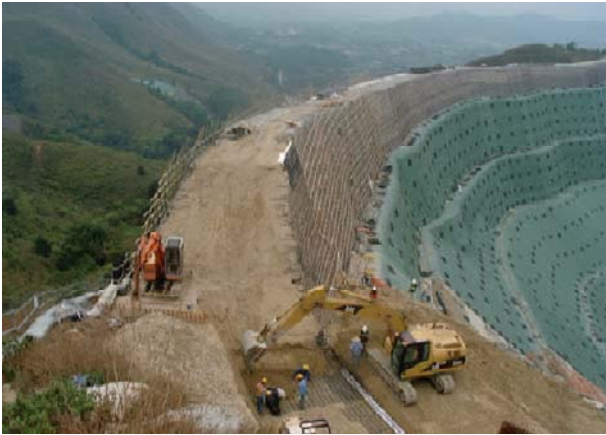
Fig. 4 The embankment nearing completion
