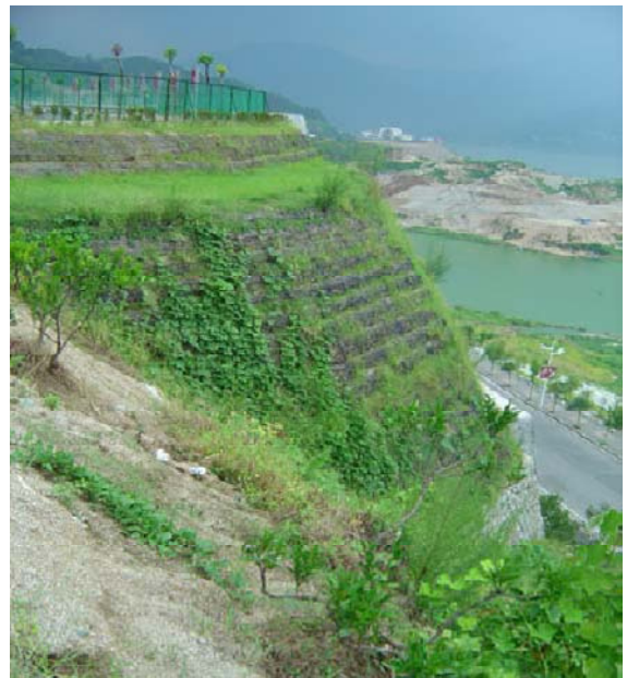
Fig. 4 Completed geogrid reinforced soilretaining wall
