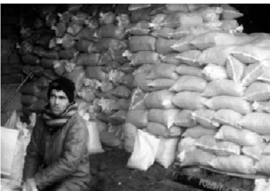
Fig. 2 Sacks containing vegetal soil and seeds to form the face of the walls
