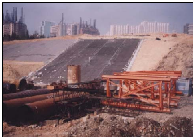
Picture 3 Earthwork capping geosynthetics
