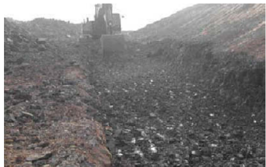
Photo 1 Treatment of basement
