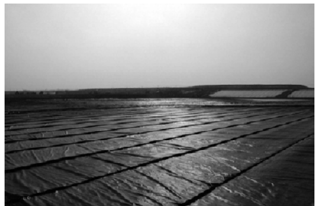
Fig. 6 Leachate filter geotextile laid out and sewn together for the Laogang Municipal Solid Waste Landfill Project Phase 4
