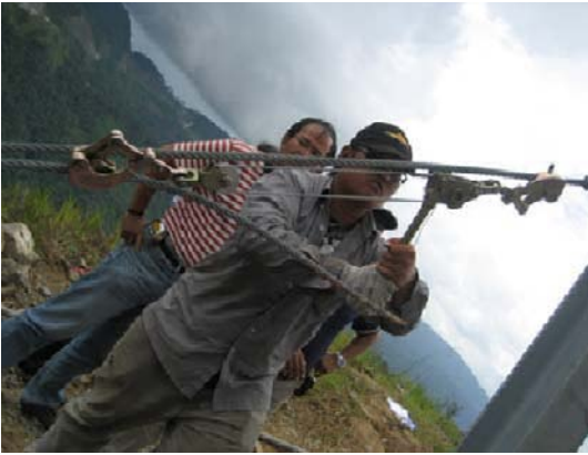
Photo 5 A “monkey wrench” being used for tensioning the diagonal wire ropes
