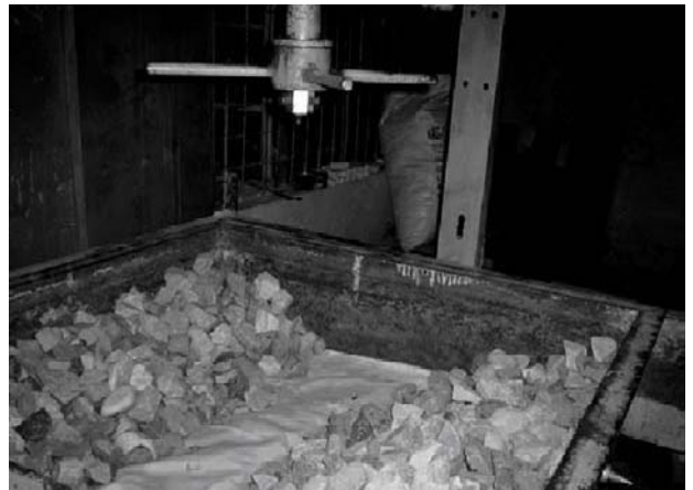
Fig. 4 Geo-synthetic placed beneath the ballast and over the sand bed
