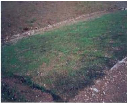
Photo 2 Slope Protection with Geomat and Artificial Grass
