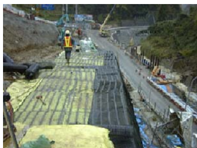
Fig. 6 Construction processes for soilbag walls
