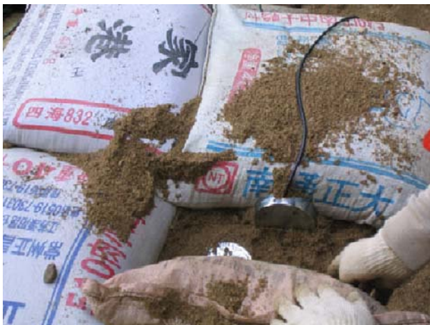
(b) Installation of earth pressure transducer
