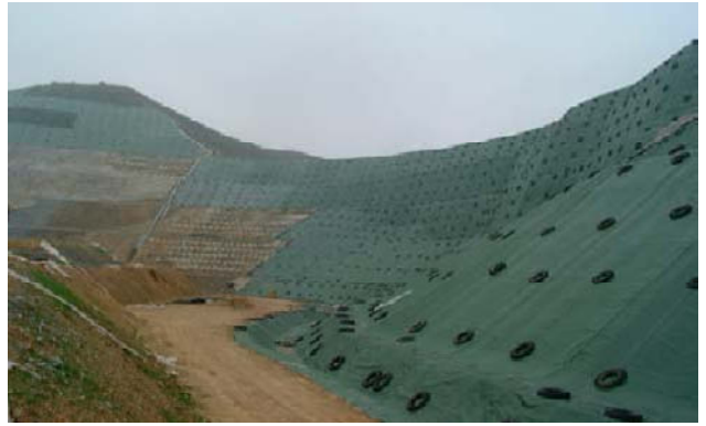
Fig. 6 Completed reinforced fill embankment on the side facing away from the waste
