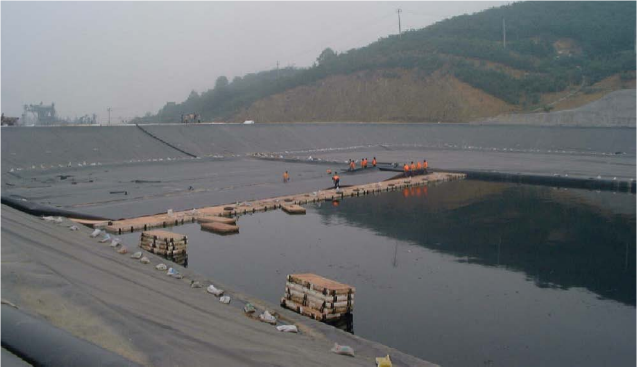
Fig. 4 Use of pontoon to deploy and seam panels
