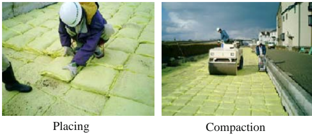
Fig. 7 Laying works
