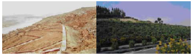
Photo 5 Comparison of untreated treated cut slope from K138+420 to K138+820
