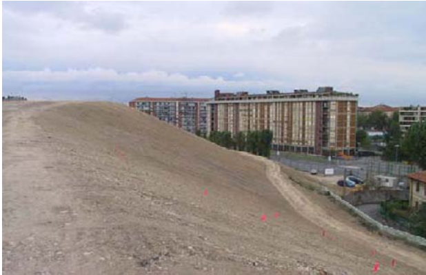
Fig. 4 View of the landfill before the beginning of the works related to the capping system
