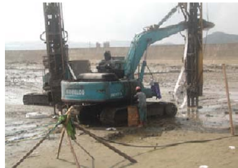
Fig. 1 Draining board installation
