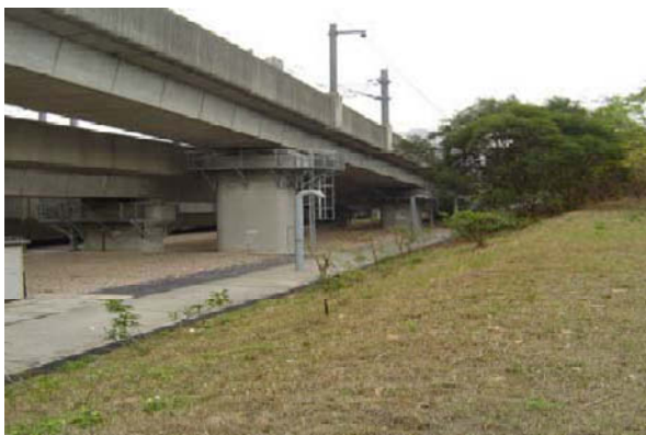
Picture 8 Vegetation on fill slope along the viaduct (1)
