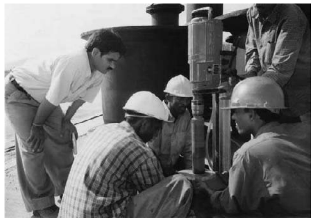
Fig. 15 Core cutting of fascia unit in preparation for concrete compressive strength test for the NH5, Dharmavaram-Tuni Package
