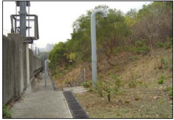
Picture 9 Vegetation on fill slope along the viaduct (2)
