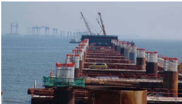
Fig. 4 Bridge construction using the trestle on the sea
