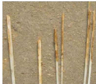
Fig. 2 The site photo of the GFRP anchor
