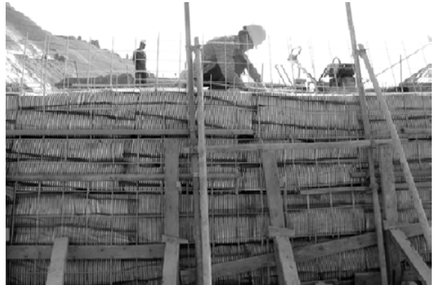
Fig. 1 Geogrid wrap around arrangement.
