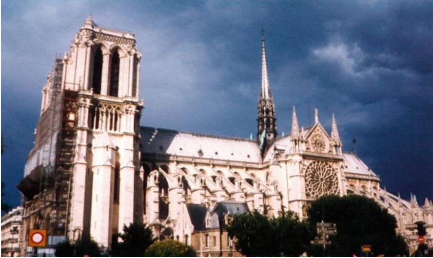
Fig. 7.6 Photo of flying buttresses utilized at Notre Dame cathedral in Paris
