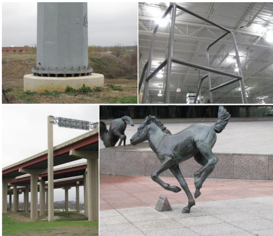
Fig. 5.5 Examples of fixed beam connections. Clockwise from top left: Connection for a large (30 m tall) highway high mast light showing 1 m diameter base; Welded connections on a portable ladder; Bronze statue of a colt showing front right leg used as a cantilever (from the bronze sculpture entitled “Mustangs at Las Colinas” by artist Robert Glen located at Williams Square in Irving, Texas); and Field of large concrete cantilevered beam–columns at a highway interchange
