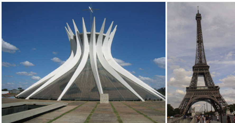
Fig. 5.2 Modern structures constructed with beams: The Cathedral of Brasilia by Oscar Niemeyer; The Eiffel Tower by Gustav Eiffel
