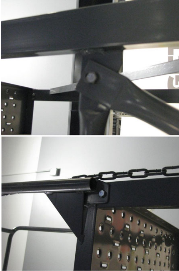
Fig. 5.4 Examples of pinned beam connections
