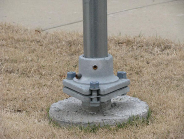
Fig. 7.9 Photo of base support system for a highway sign designed to fail if impacted by a vehicle
