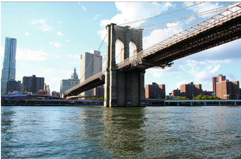
Fig. 6.3 Photo of the Brooklyn Bridge
