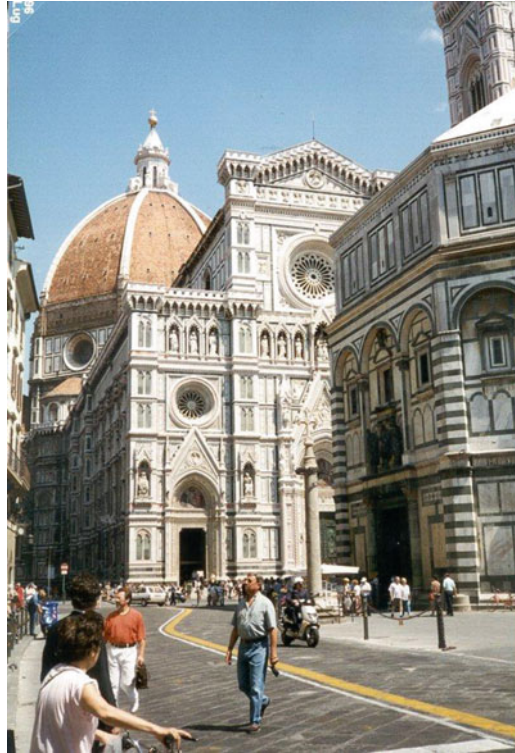
Fig. 1.6 Photo of the Brunelleschi dome in Florence
