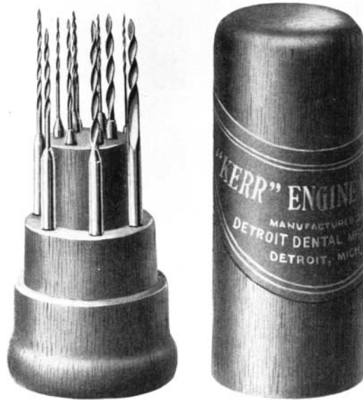
Figure 10-32 Historical illustration of Kerr Engine Drills, circa 1912. The shape of the drills resembles present-day K-style reamers. Made of carbon steel, they were probably safe to use in straight canals with a slow, treadle-type, foot-powered handpiece. (Courtesy of Kerr Dental Manufacturing Co., 1912 catalog.)
