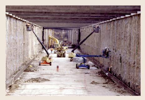
**FIGURE:** Mid-corridor track construction (image courtesy of the Alameda Corridor Transportation Authority).
