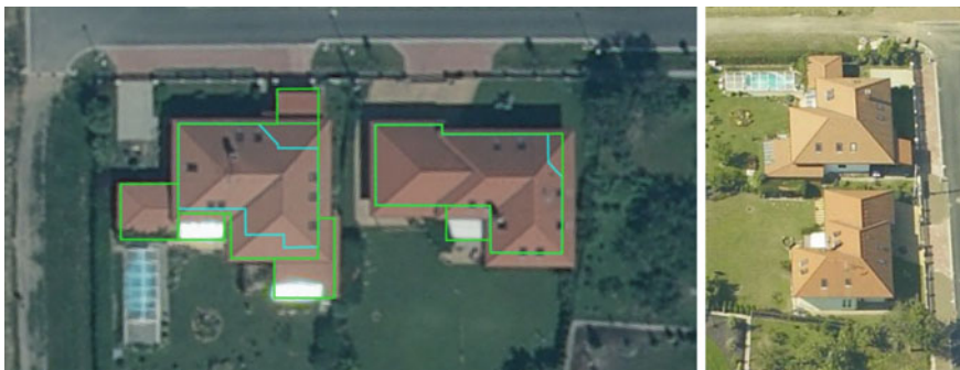
Fig. 1 Left Orthoimage of two buildings with roof overhangs ( green line ) over the outer walls ( cyan line ). Right Oblique image of the same buildings taken from the east
