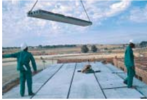
Figure 1: Erection of hollow core slabs
