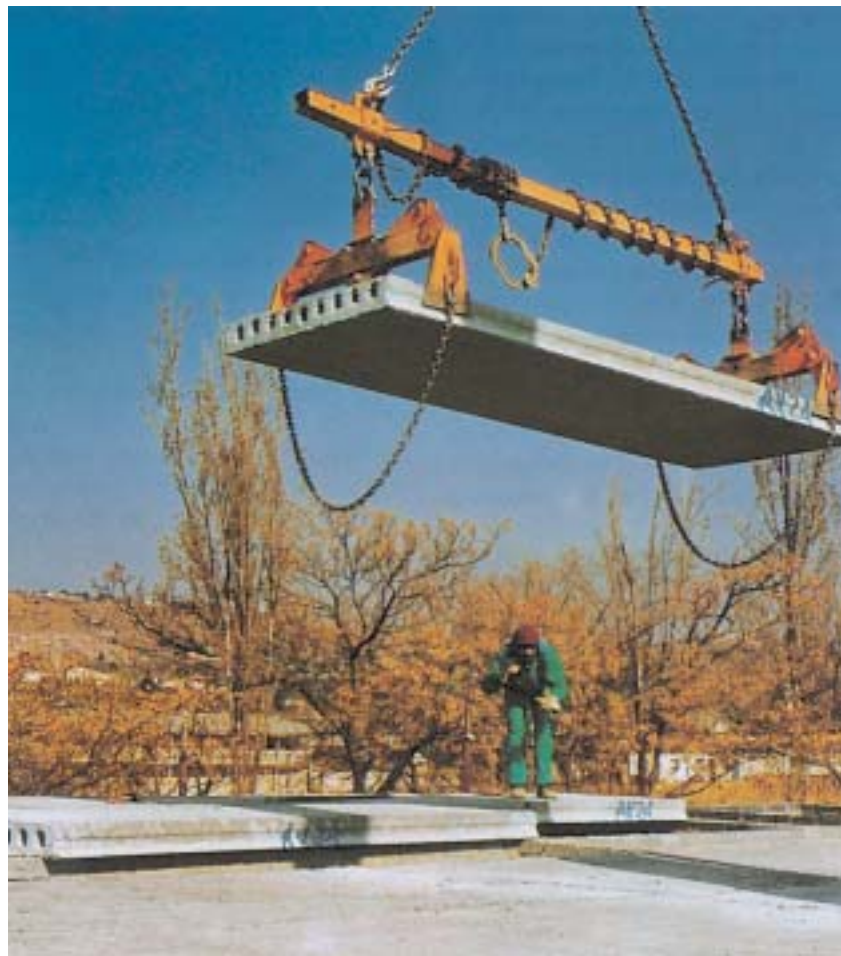
Fig 3: Hollow core slab being hoisted into position
