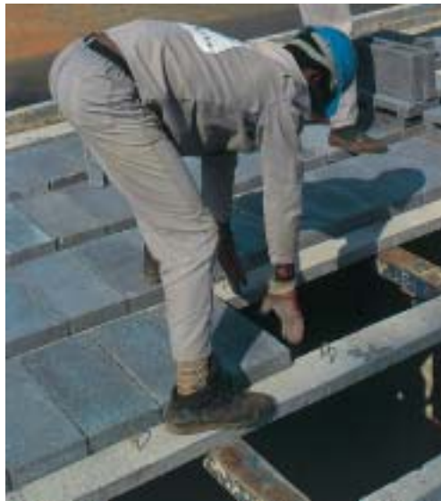
Figure 22: Placing blocks into position.
