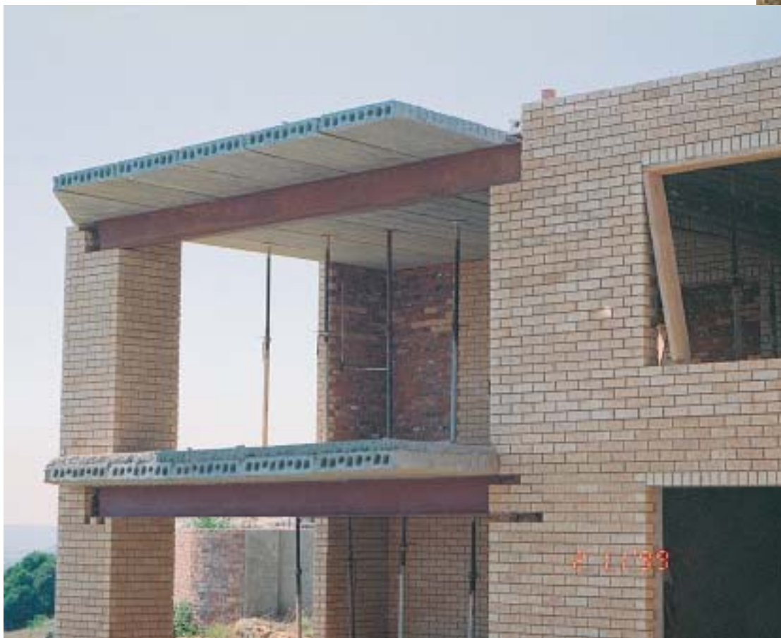
Figure 30 and 31: Steel beams used over large openings
