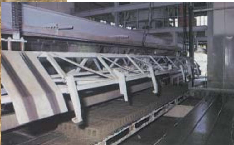
Figure 9: Manufacture of reinforced hollow core slabs.
