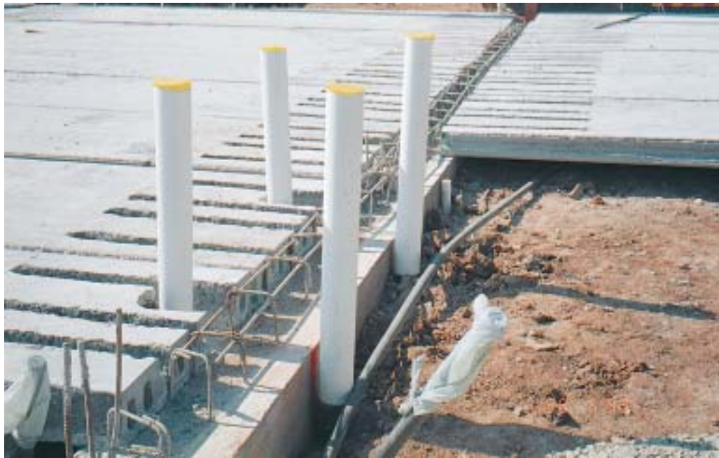
Figure 12: Prestressed hollow core used as a suspended ground floor slab
