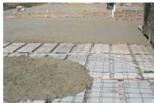
Figure 39: Casting concrete.
