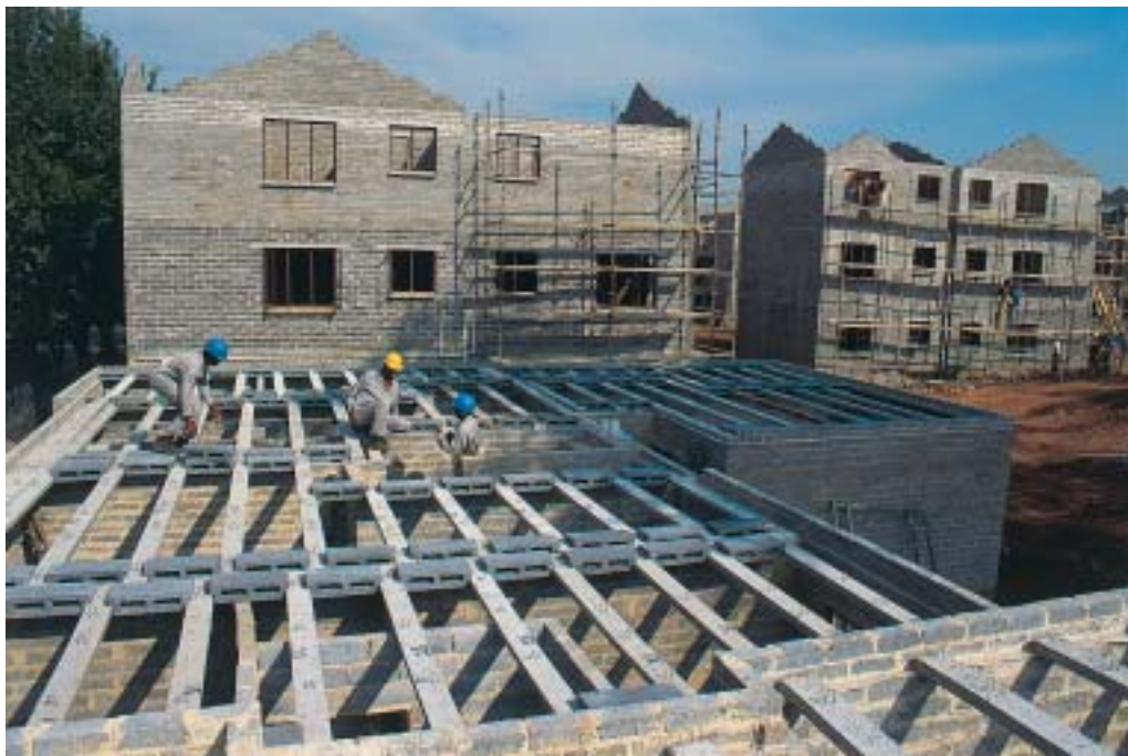
Figure 2: Prestressed beam and block slab under construction
