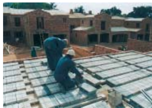
Figure 38: Mesh placed over blocks.
