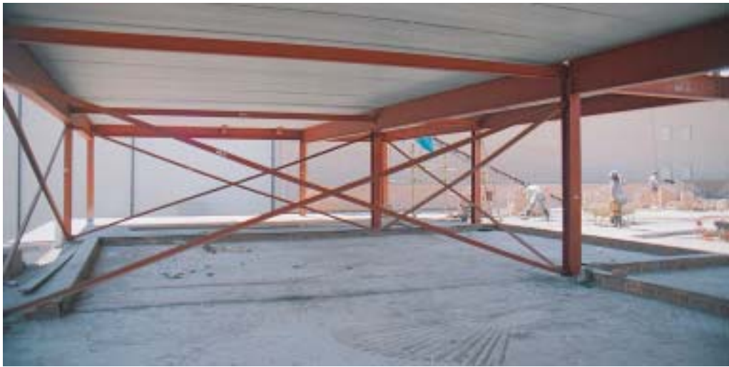
Figure 5: Use of hollow core slab on steel frame.
