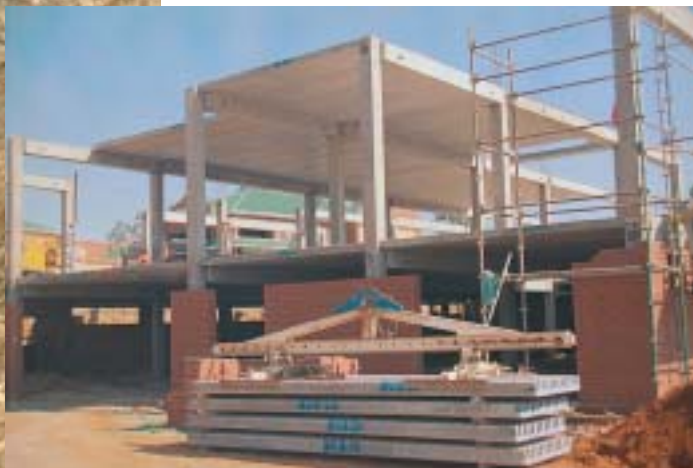
Figure 29: Precast hollow core slabs and precast beams erected on in situ columns.
