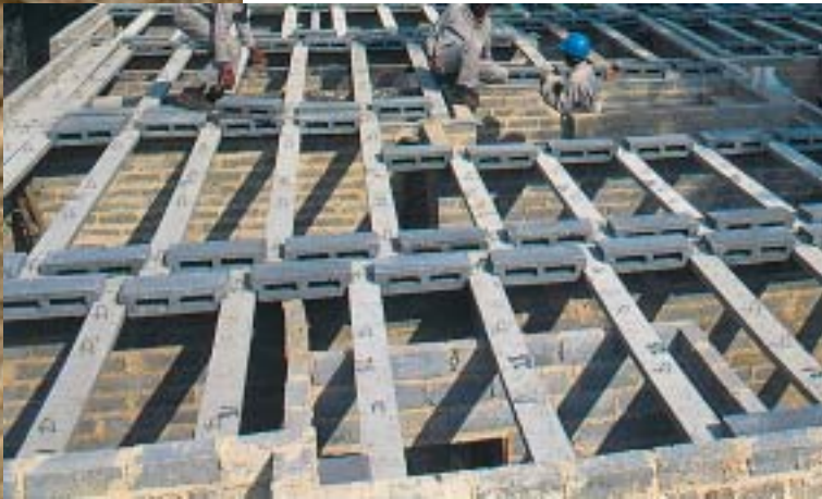
Figure 19: End filler blocks placed to determine correct beam spacing.
