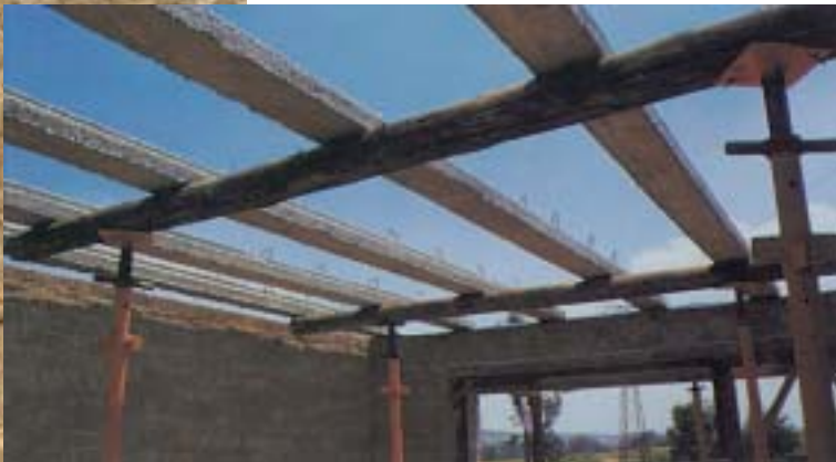
Figure 20: Prestressed beams in place with support.
