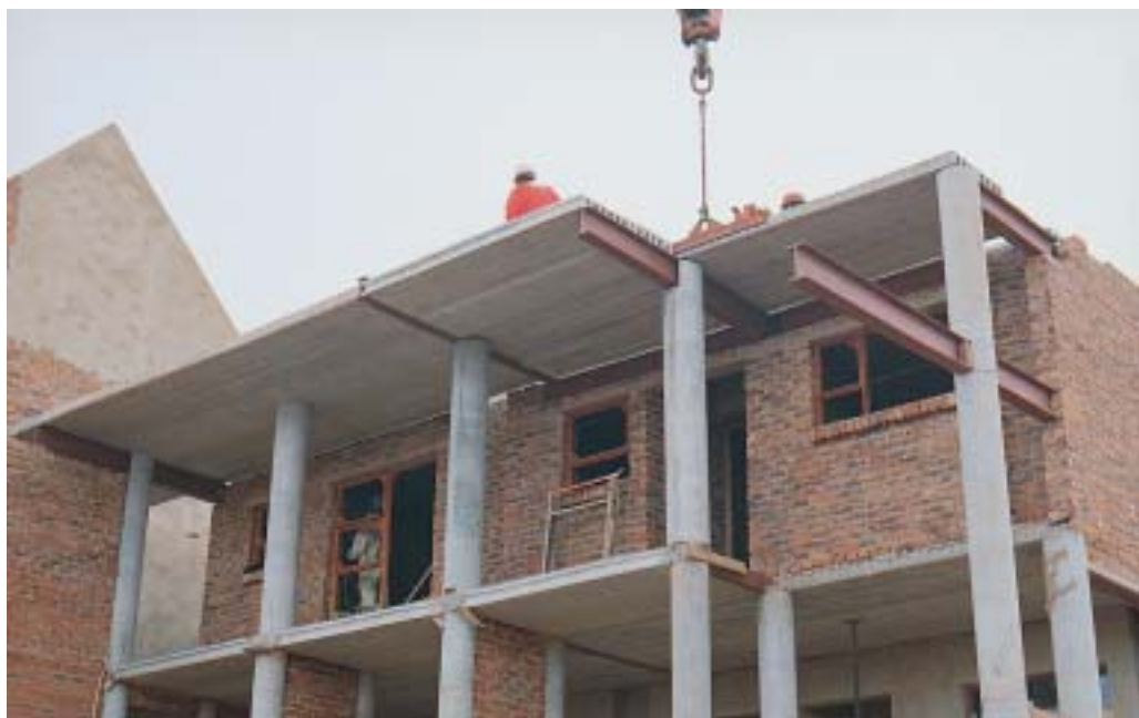
Figure 13: Hollow core slab
