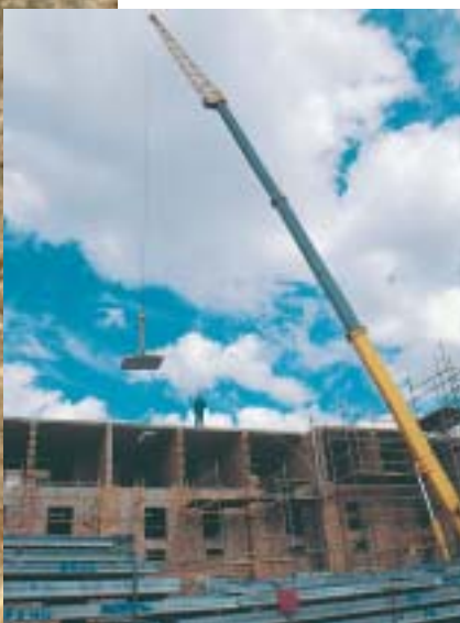
Figure 34 & 35: Hoisting slabs into position.
