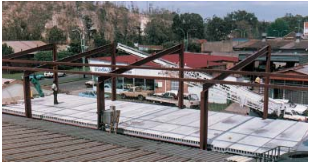
Figure 16: Hollow core slab on steel frame. Note omission of purlins for crane access.
