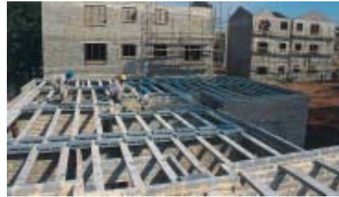
Figure 36: Setting out of beams.
