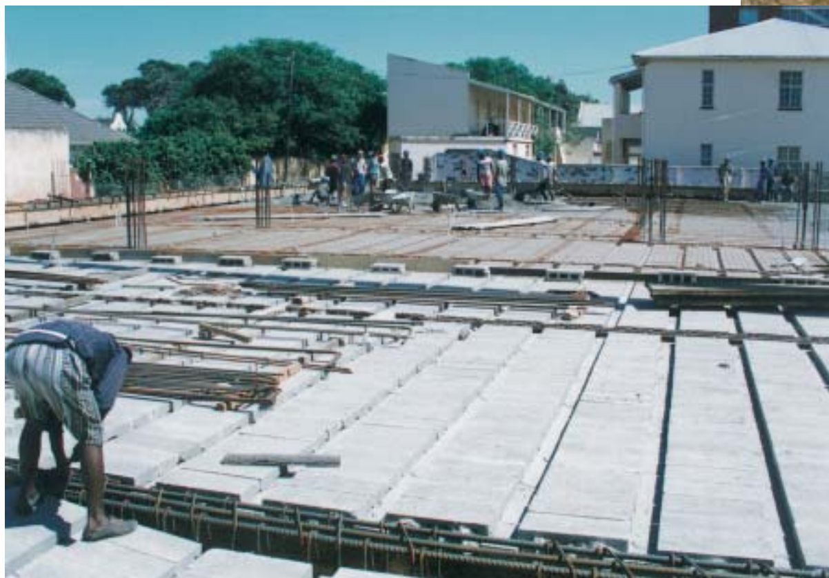
Figure 26: Preparing and casting of a precast beam and block slab in progress.
