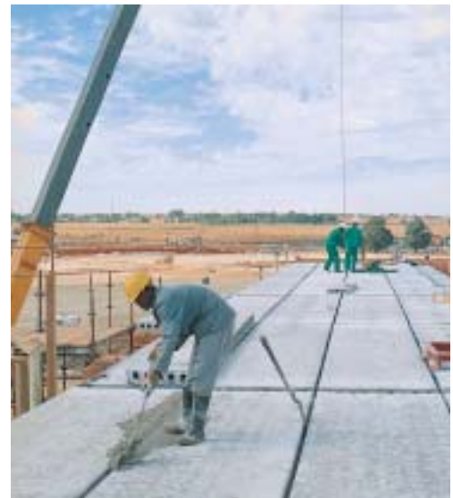
Figure 33: Grouting joint between hollow core slabs.
