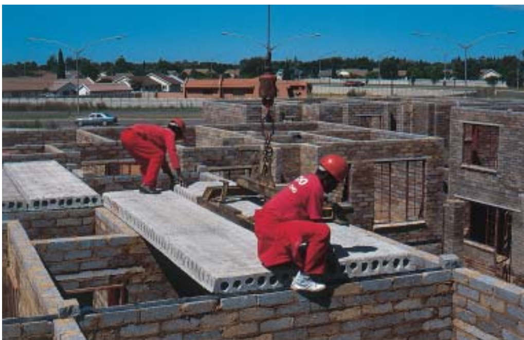
Figure 15: Hollow core slab, for a townhouse complex.
