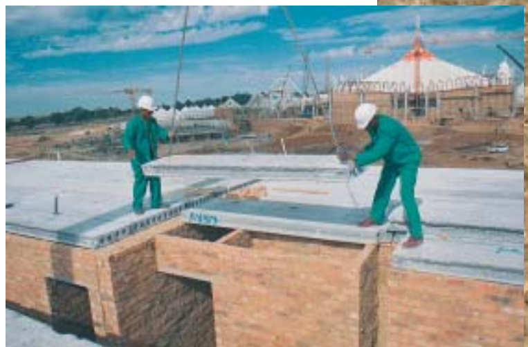
Figure 11: Hollow core slab being hoisted into position direct from the delivery vehicle by mobile crane.
