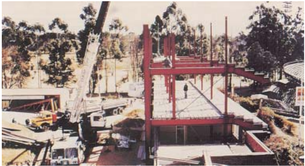
Figure 17: Hollow core slabs used on seating areas of the Wanderers grandstand.
