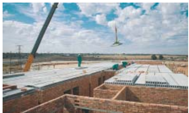
Figure 34 & 35: Hoisting slabs into position.
