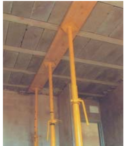
Figure 21: The soffit of a beam and block slab.
