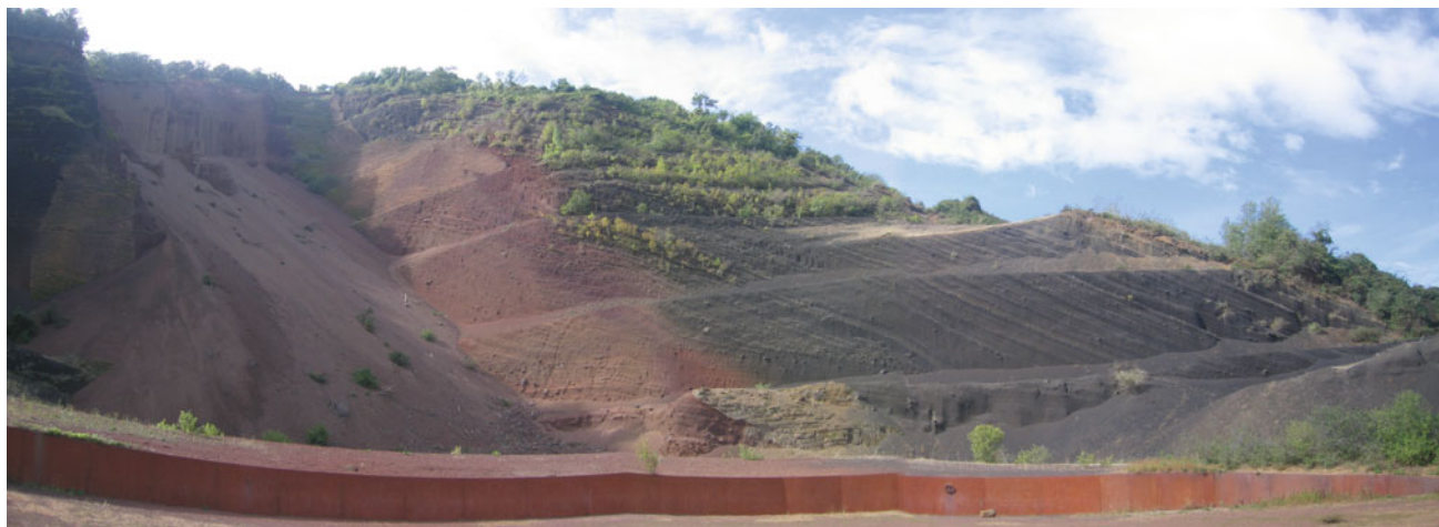
Fig. 1.13 Restoring the landscape inside the volcano Croscat. Source Catalan Landscape Observatory
