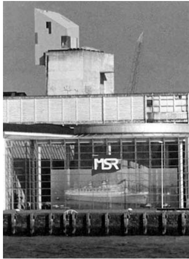
Figure 11.9 The Las Palmas building in Rotterdam, a roof 'Parasite'.
