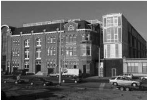
Figure 11.10 Looiershof, showing the existing building facade, new extension and roof reuse. (Source: Hulshof Architects.)
