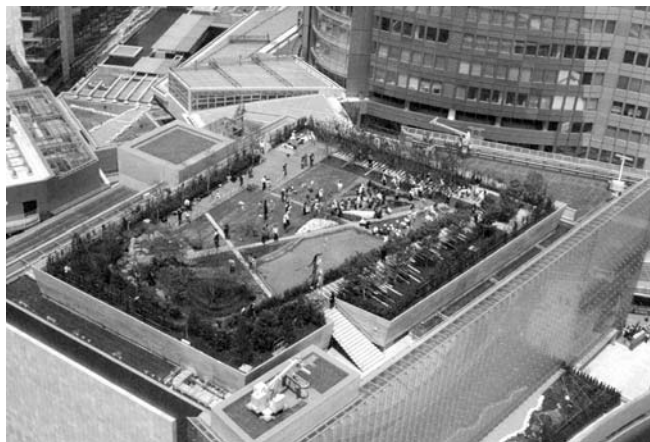
Figure C.30 A 'sky garden' at Roppongi Hills, Tokyo. (Source: Mori Building Co., Ltd.)
