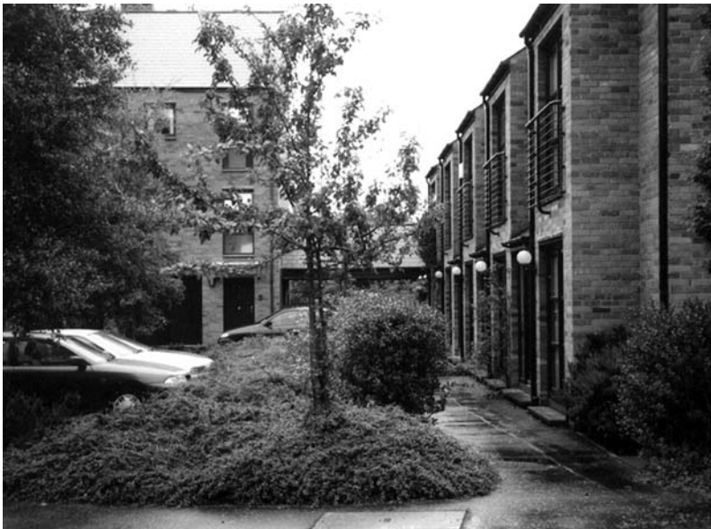
Figure 15.15 Three-storey town houses in Northern Ireland, thought by many to be too high a density. (Source: Mike Jenks.)
