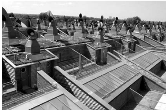
Figure C.23 Using the roofs to give private gardens in a high-density development. (Source: www.zedfactory.com )
