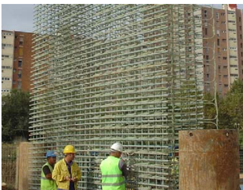
Figure 1-3: Soft eye FRP reinforcement
