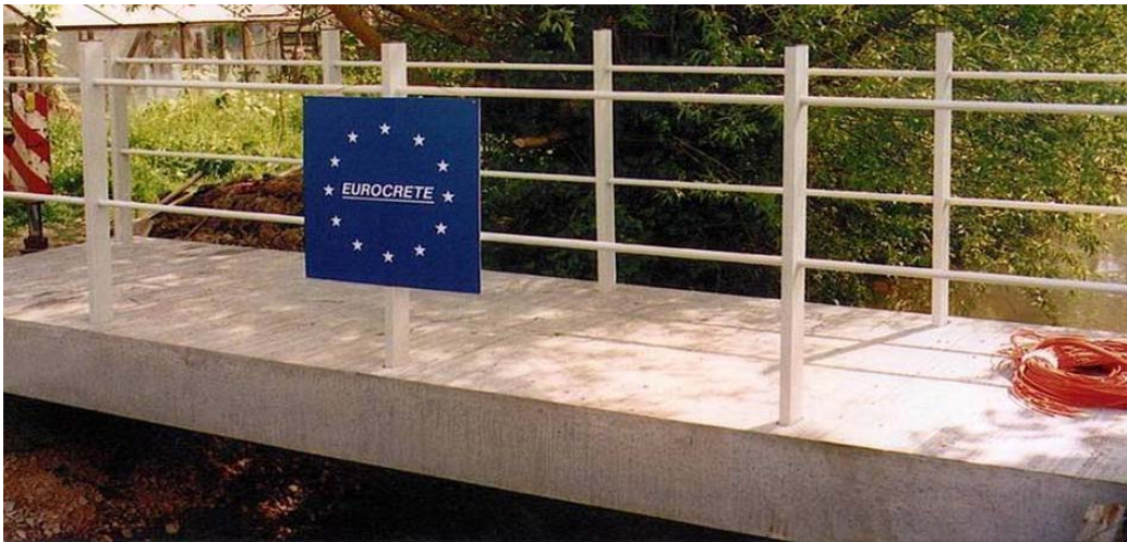
Figure 1-1: The first concrete footbridge in Europe with only FRP reinforcement (EUROCRETE project)
