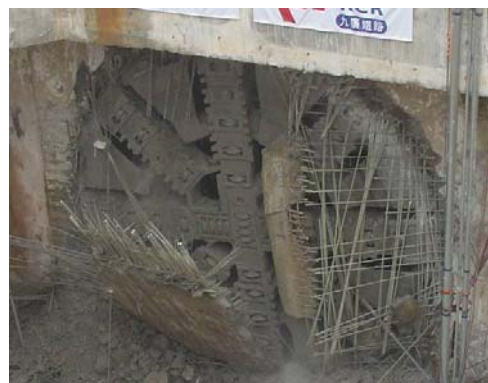
Figure 1-3: Soft eye FRP reinforcement
