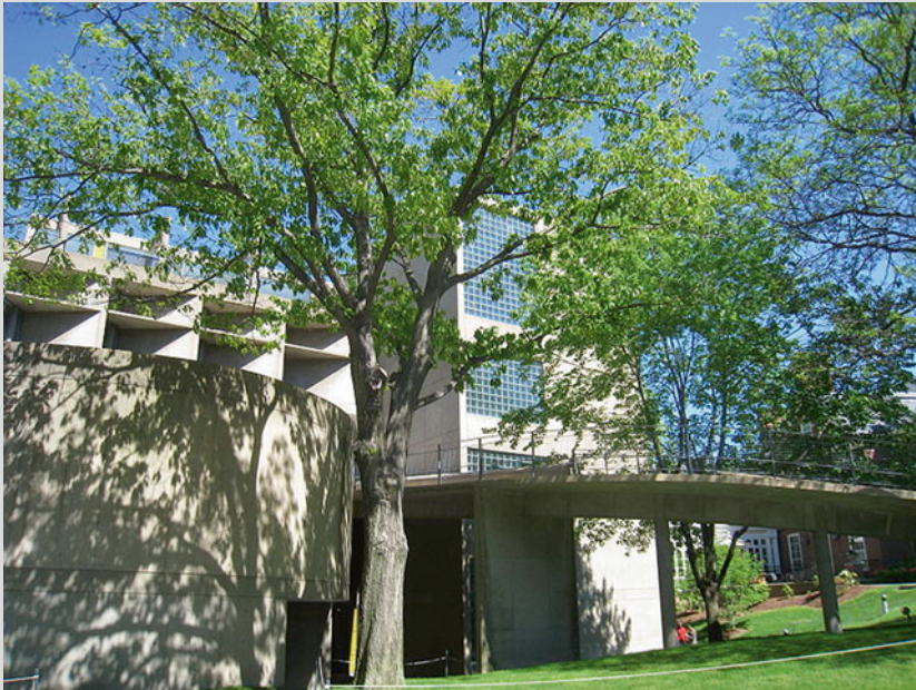
Fig. 9.1 The Carpenter Center, Harvard University, Cambridge, MA, USA. (Notice the brise soleil and the glazed windows) (Source: Wikimedia.org. http://commons.wikimedia.org/wiki/File:Carpenter_Center_Harvard_University.jpg )
