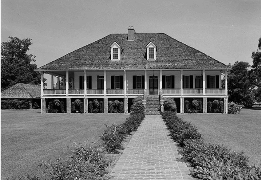
Fig. 2.3 Plantation house in colonial Louisiana in vintage ‘French colonial’ architecture. Notice the raised basement, full-length porch, exterior stairs, steep hipped roof with dormer and French doors (Source: Wikimedia.org. http://commons.m.wikimedia.org/wiki/File:Oaklawn_Plantation_house.jpg )
