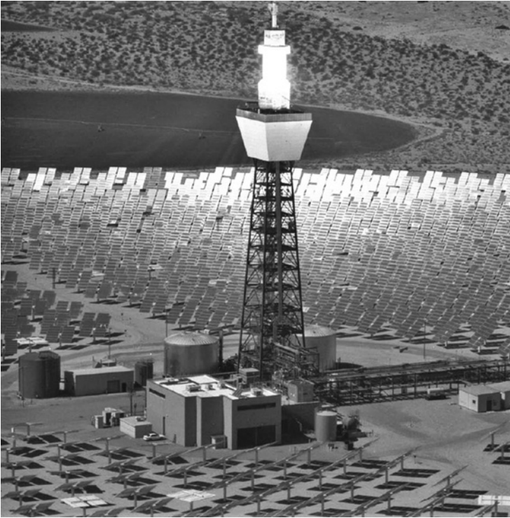
Figure 28.3 Solar power tower power plant. Source: Reproduced with permission of U.S. Department of Energy, Waste Isolation Pilot Plant, http://www.wipp.energy.gov/science/energy/powertower.htm .
