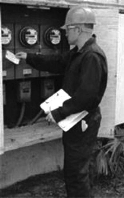
Figure 1.6 Photo of typical arc flash protection PPE. Source: Reproduced with permission of OSHA.
