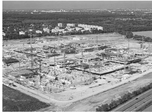
Figure 3. View of the construction site of the BauVOGrid reference project ARGE Campeon : The Infineon Headquarters at Neubiberg near Munich – gross area 250000 m 3 , total costs 240 MEuro, constr. time 18 months, 140 sublocations to be managed.
