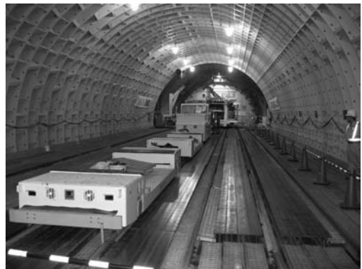
Figure 1. A photograph of a shield tunnel under construction in Tokyo.
