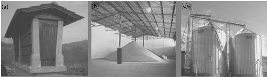
FIGURE 2.2 Different types of cereal storage: (a) traditional, (b) cellar storage, and (c) silos.
