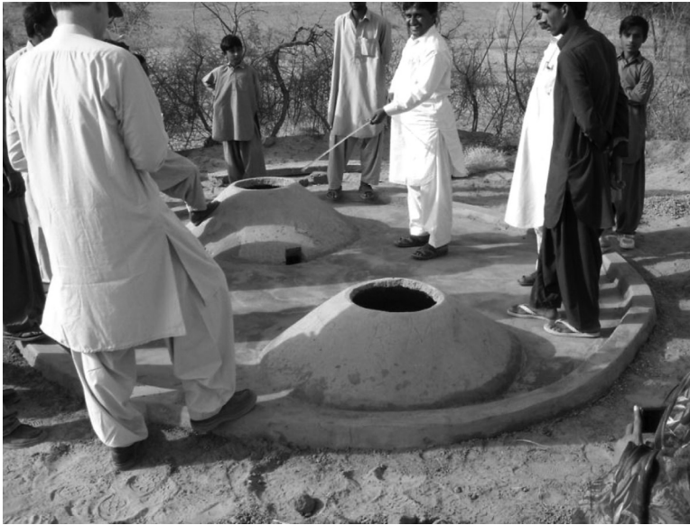
FIGURE 25.17 Water tank at Thar and Cholistan Deserts, Sind.
