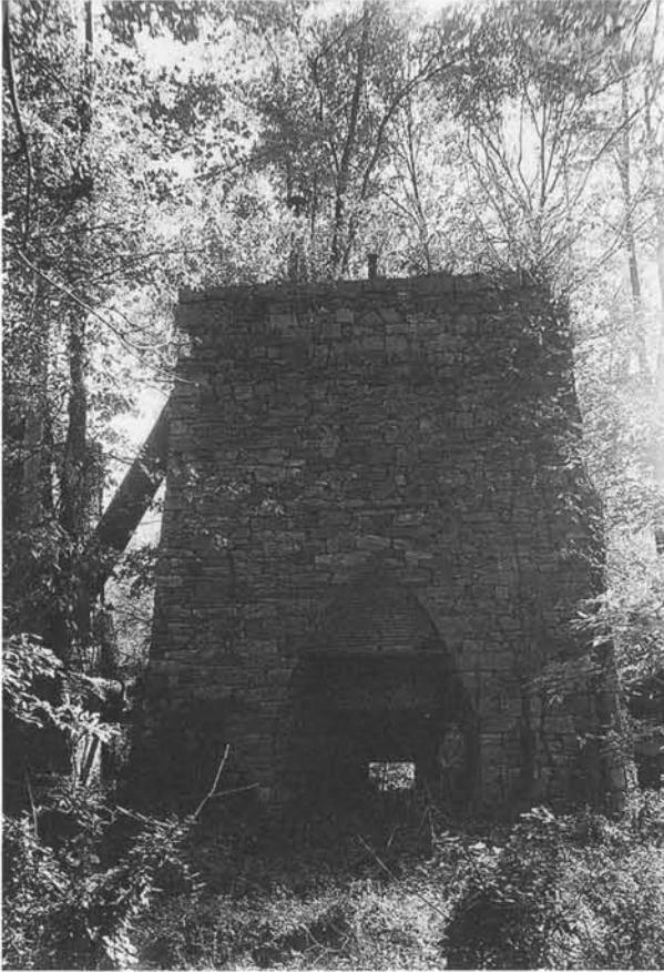
This massive blast furnace was part of the Principio Iron Works in Maryland, one of colonial America's largest iron enterprises. Courtesy of the Library of Congress.
