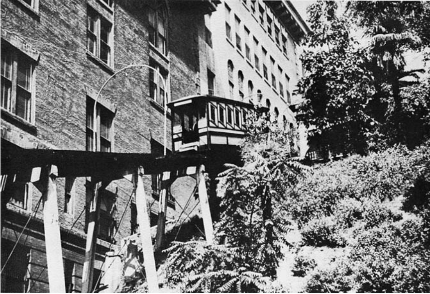
Figure 2.6: Funiculars like the Mt. Lowe line were built in several cities, including Cincinnati, Duluth, and Pittsburgh, and on the Palisades across the Hudson River from Manhattan. Two Pittsburgh funiculars remain in operation to this day. In Los Angeles, Angels Flight operated between 1901 and 1969, climbing a 33 percent grade for 335 feet to an increasingly seedy neighborhood called Bunker Hill. Its noir ambience was woven into the popular imagination through the movies. Jimmy Stewart, Lon Chaney, Ann Sheridan, and William Holden all had their dramatic moments around Angels Flight. (Author's photo)
