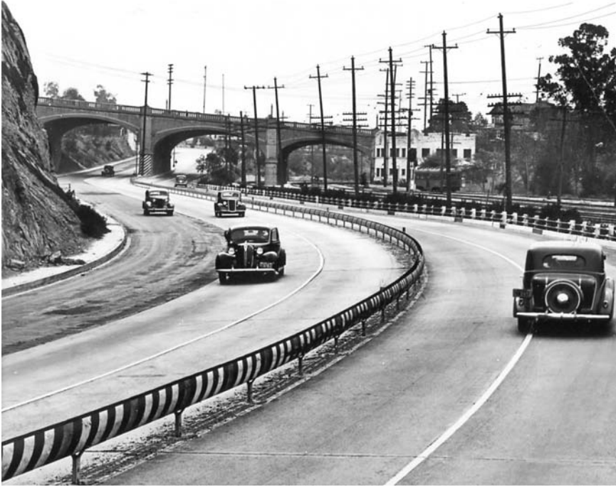
Figure 4.7: One of the early limited-access highway projects in the United States was this stretch of Ramona Blvd., east of downtown Los Angeles, which looks invitingly free of congestion in this 1937 photo. After World War II, passenger service on the Pacific Electric Railway line at the right would be abandoned, while Ramona Blvd. was transformed into the San Bernardino Freeway, now Interstate 10. (Courtesy Automobile Club of Southern California Archives)
