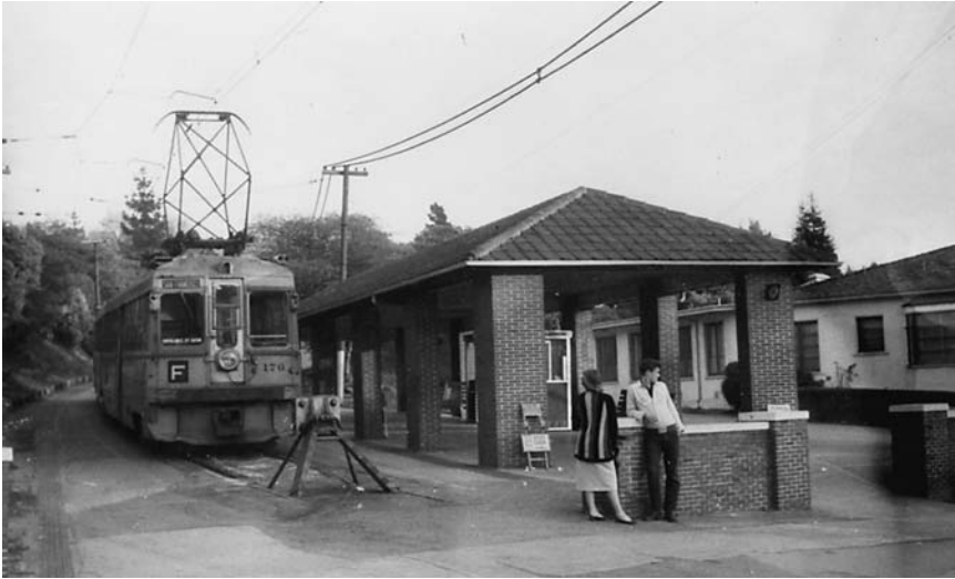
Figure 4.6: When the Bay Area Rapid Transit (BART) began running electric trains through its transbay tunnel, it was in essence reviving the Key System's service which connected San Francisco with the East Bay via the Bay Bridge beginning in 1939. Looking quite modern, here is the station at the end of the Key System line near the University of California just before the end in 1958, when tracks on the bridge were removed to make way for additional lanes of automotive traffic. (Author's photo)
