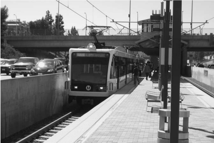
Figure I.1: The light rail line connecting Los Angeles and the San Gabriel Valley follows a former Santa Fe Railway right-of-way for almost its entire length; here, in Pasadena, it runs in the median of Interstate 210. There are trains rather than single cars, and passengers step directly aboard from high-level platforms. This is like rapid transit and unlike a typical streetcar line. The major similarity is the power pickup overhead (by means of a double-hinged device called a “pantograph,” a modernized version of a trolley pole) whereas rapid transit utilizes an electrified third rail next to the tracks. Such a third rail would not be feasible with this light rail line, or any other, because in places tracks are embedded in public streets and would put people in harm’s way. (Lee Furon photo, author’s collection)
