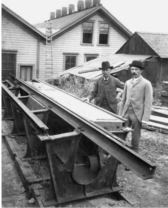
Figure 1.6: Frederick Wood and John Fowler, superintendent and general manager of the Temple Street line, show off a cross-section of track and conduit, much more substantial (and costly) than the original Clay Street line. In 1892, the same year the photo was taken, Wood (at left) published a technical treatise titled On the Temple Street Cable Railway in Los Angeles, California, with illustrations of numerous refinements that he and Fowler had devised, including a double-jaw side grip that obviated the need for a turntable at each end of the line, as in San Francisco. Alas, no matter how ingenious these two men may have been about mechanical matters, cable propulsion was on the verge of being rendered obsolete by electricity. (Security First National Bank photo, author's collection)
