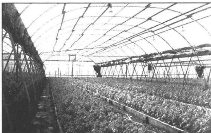
Fig. 2.8 Interior view of interlocking ridge and furrow type Quonset greenhouse.
