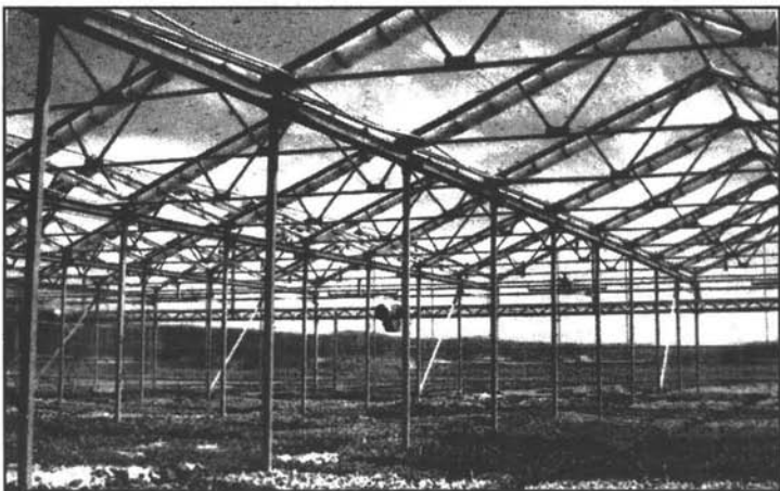
Fig. 5.3 Gutter-connected retractable roof polyethylene greenhouse.
