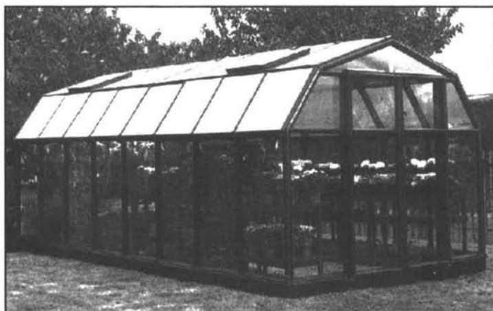
Fig. 8.1 Fiberglass-reinforced plastic rigid panel greenhouse.
