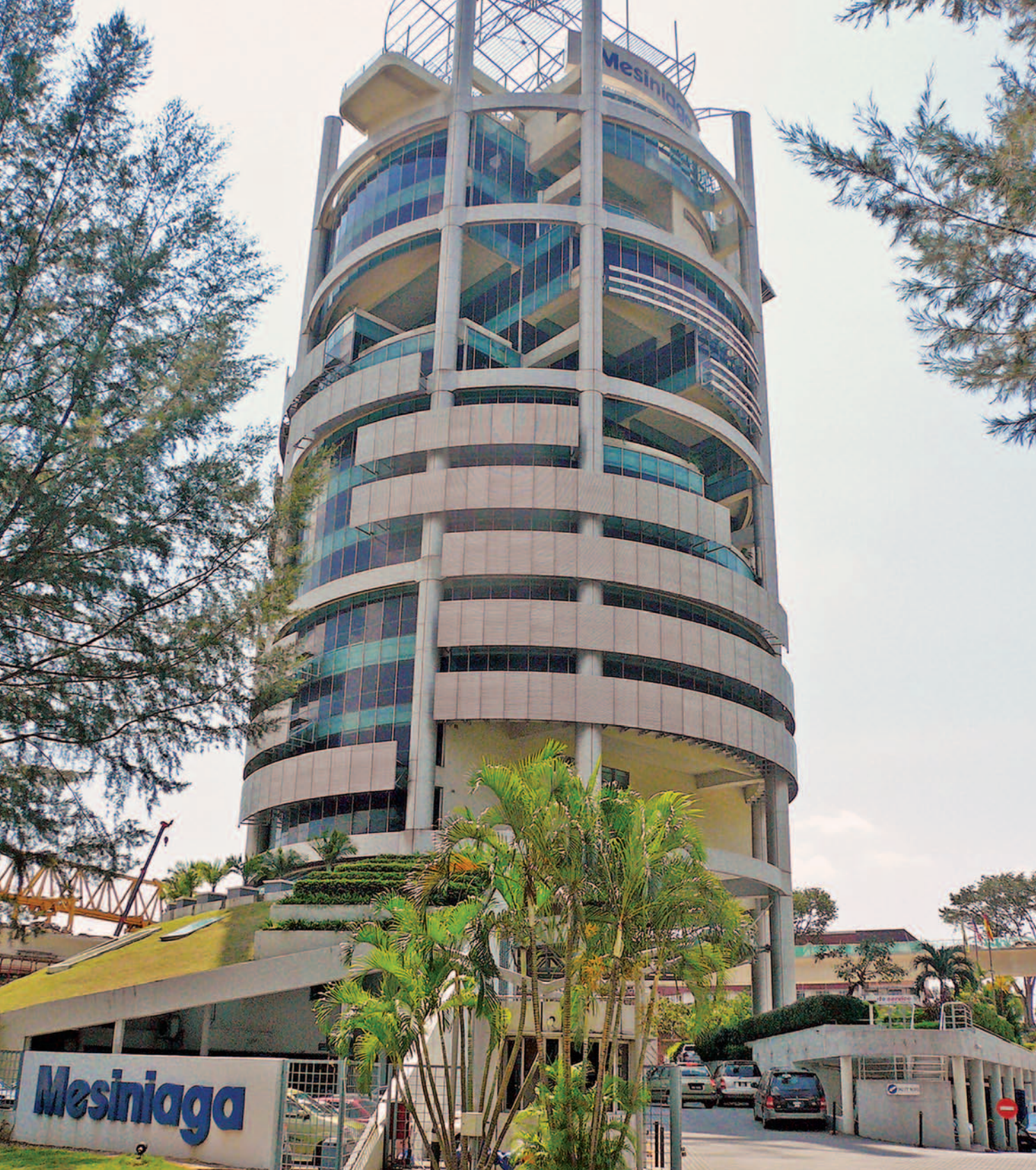
Menara Mesiniaga looks different than most other skyscrapers. And it provides a healthy and eco-friendly working environment.
