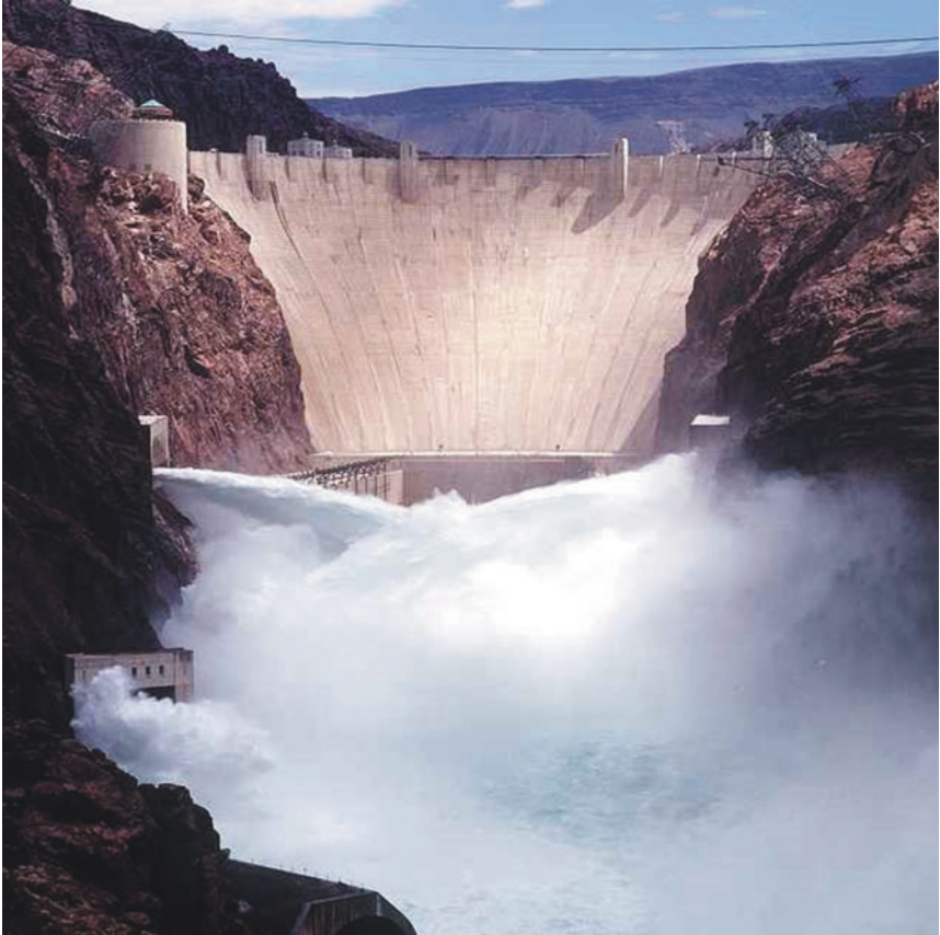
Fig. 6.2 Hoover Dam with downstream water releases
