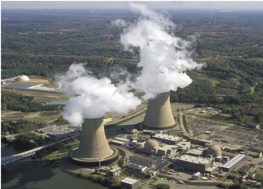
Fig. 2.3 Aerial photo of Beaver Valley Power Station in Pennsylvania, showing evaporation loss from the large cooling towers
