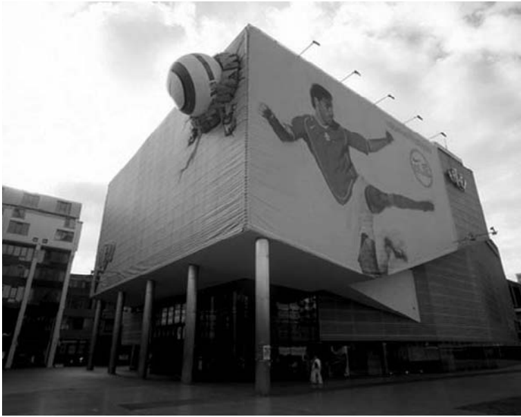
Fig 3: Temporary façade [Vertical Vision, www.verticalvision.com ]
