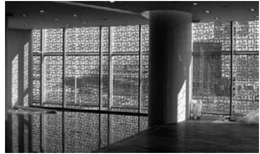
Fig. 34 Office Tower at the Burjuman Centre in Dubai. Panels in middle of façade.
