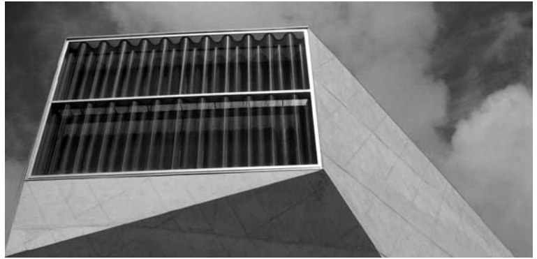
Fig. 7. The façade of the Casa da Musica; corrugated glass and white concrete: an unexpected match.
