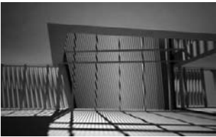
Fig. 36-38 above and below: Office building in hot climate with vertically-set louvers that move to change opacity with varying requirements for shading, daylight and natural ventilation.
