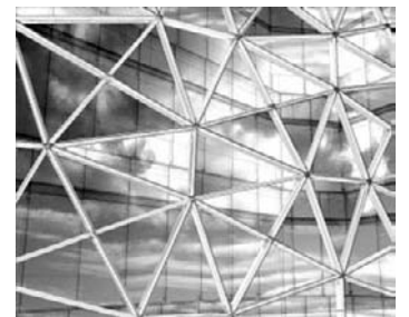
Fig. 10 above: The form of the building is formed by twisting the outside form of the building and curving each façade by a different amount. This creates a complex form which can be constructed from repeated panel types.
