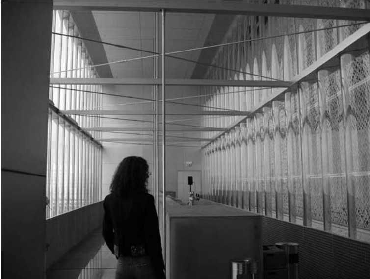
Fig. 5. In between the two corrugated glass walls a bar was installed, made of glass, of course. Above hang the trusses that take up the wind load on the façade.
