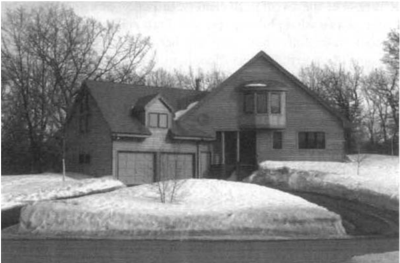
The facade of this modest Minnesota house by Dale Mulfinger takes special care to convey values important to a suburban culture: the garage, the ceremonial front door, and the window of the master bedroom.
