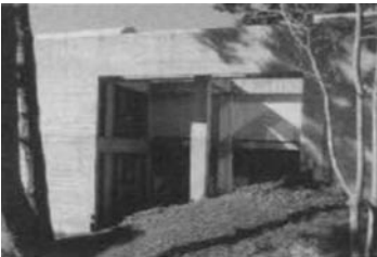
Land, air, and sky meet in the courtyard of the Wall House. Photograph courtesy of Tadao Ando.
