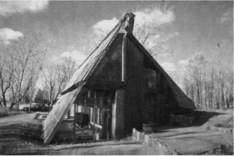
Oroborous, a research project of the University of Minnesota, was designed to be heated with solar energy and electrified by a windmill. A clivus multrum processed human waste into the soil.
