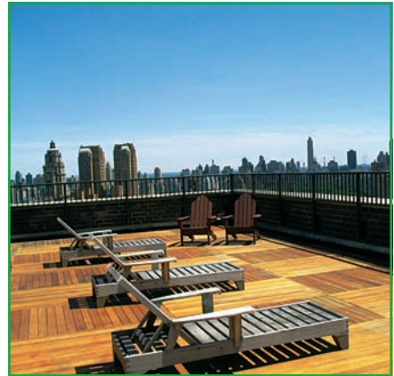
People have become accustomed to a variety of products made from recycled plastic. This deck and the furniture are made from plastic lumber. Plastic lumber comes in a variety of grades, colors, textures, and weights. ( Plastic Lumber Yard )
