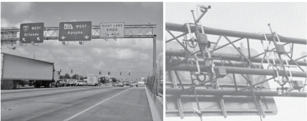
Figure 8.12 SR-436 surface street evaluation site.
