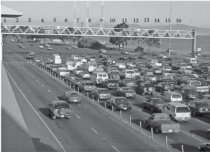
Figure 3.12 Mainline metering of vehicles heading west onto the San Francisco–Oakland Bay Bridge. (From Caltrans District 4, Oakland CA.)
