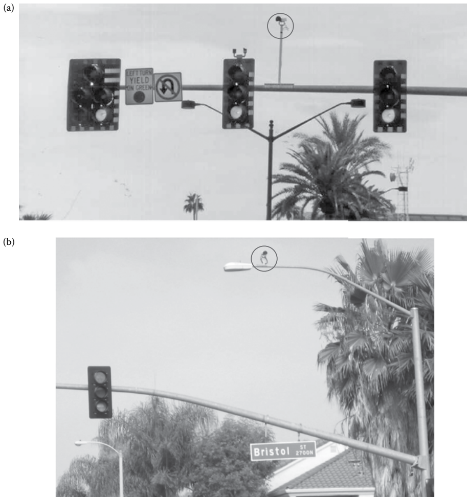
Figure 3.4 Camera mounting options for VDSs deployed at signalized intersections. (a) Camera mounted on signal mast arm over center of monitored lanes. (b) Camera mounted higher on luminaire off to side of monitored lanes. (From LAK.)
