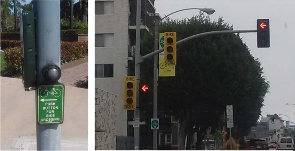
Figure 1.6 Traffic signal controls for requesting and notifying a cyclist of a green signal phase. The bike signals are highlighted with a yellow housing in the photograph on the right.
