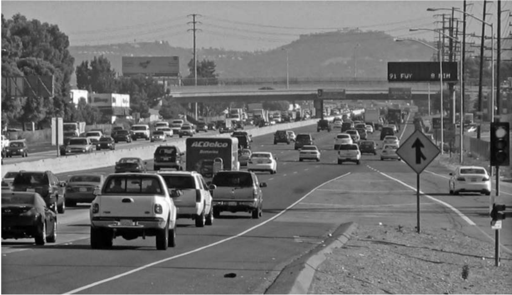
Figure 3.9 Sensors (not shown) determine travel times displayed on changeable message signs and ramp meter signal cycle times. (From LAK.)
