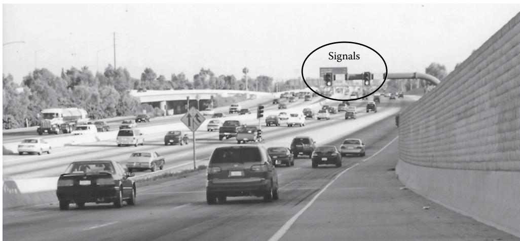
Figure 3.11 Freeway-to-freeway metering on the connector from the eastbound I-105 Freeway onto the southbound I-605 Freeway in Norwalk, CA. Meters on the two I-105 lanes allow three vehicles per lane during each green cycle to enter the four lanes of the I-605 mainline. One of the two I-105 ramp lanes continues as a fifth mainline lane. (From LAK.)
