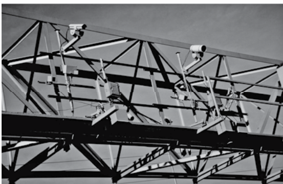
Figure 8.16 I-10 freeway sensor evaluation site near 13th Street in downtown Phoenix. Overhead sensors were mounted on the sign bridge facing approaching traffic.
