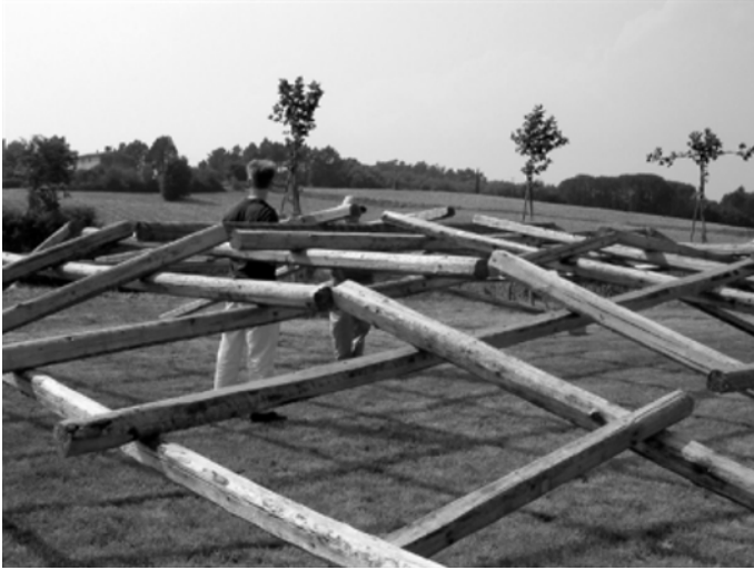
Fig. 4. First dome completed
