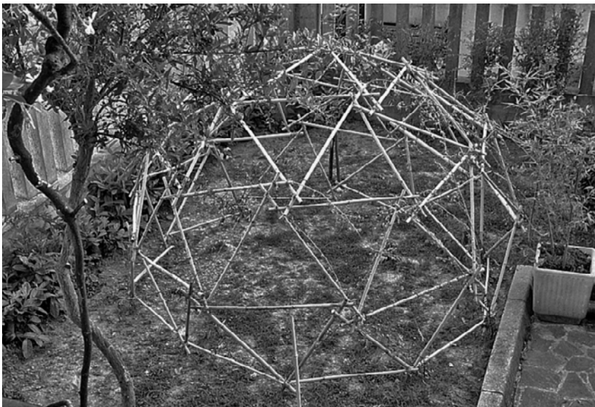
Fig. 6. Reciprocal frame in bamboo, icosahedron Alt 2v, 5/8 section of a sphere, diameter 2.92 m, maximum height 1.83 m. If covered, could be used a a shelter from the sun
