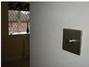
Plate 11 Rotary dimmer switches of this type can be used with GLS lamps but are not suitable for most types of compact fluorescent lamps
