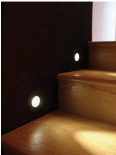
Plate 17 Some well lit stairs; low level lighting by LEDs is provided at the side of each stair tread
