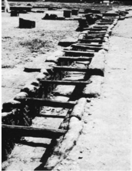
Figure 1.1 Picture of Mohenjo-Daro excavated sewer channel (Hodge, 1992).
