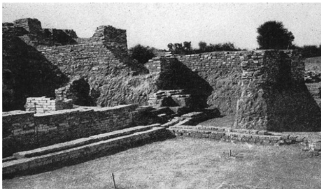
Figure 1.2 Picture of Harappan above ground sewer channel constructed of burnt brick (Kirby et al. 1956).
