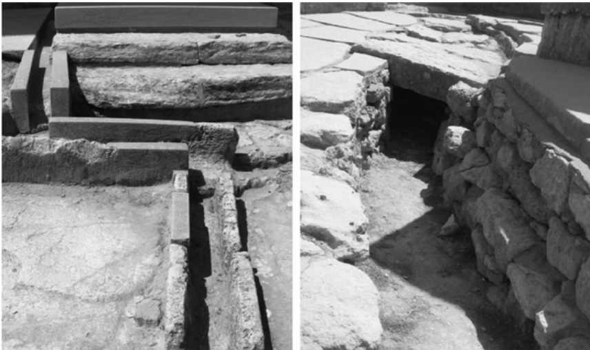
Figure 1.3 Parts of the sanitary and storm sewage systems of Knossos Palace (Lofrano & Brown, 2010).
