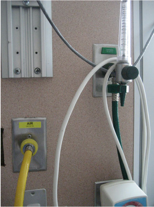
Figure 13.5. Centralized oxygen source via specific connections are often distinguished by different colors and signs.
