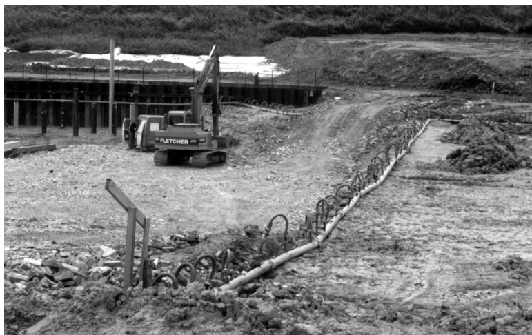
Pumping system used during construction (middle and bottom picture)
