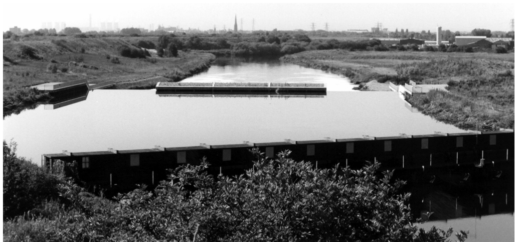
Finished weir in operation (photographs courtesy of HR Wallingford)
