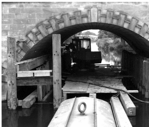
The boulders (right) were removed from the bed when pile driving was required for works to the bridge arch (photographs courtesy of Mott MacDonald)
