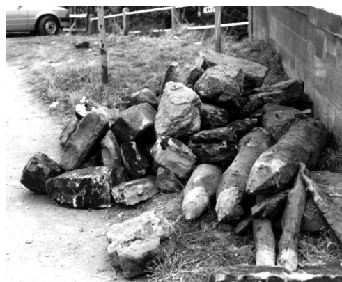
The boulders (right) were removed from the bed when pile driving was required for works to the bridge arch (photographs courtesy of Mott MacDonald)
