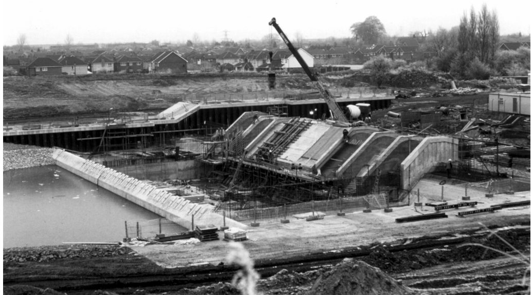
Construction of the syphon weir (downstream channel flooded)
