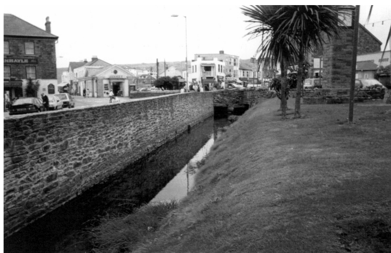
Figure A4.2. Raised river wall along Tywarnhayle Square
