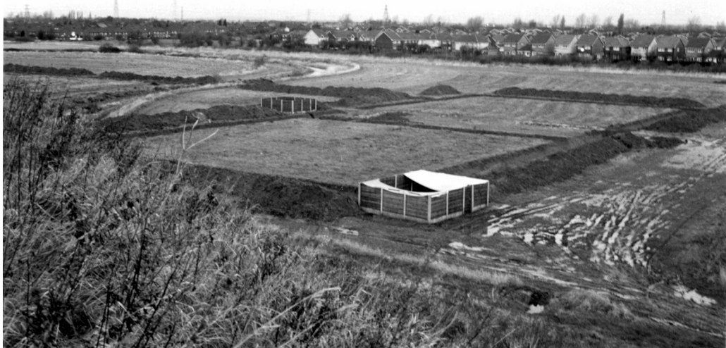
Trial pumping to develop and test drainage system
