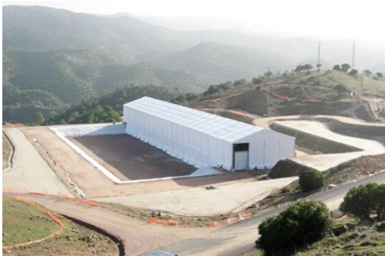
Courtesy of Enresa. Centralized VLLW disposal El Cabril (under Creative Commons License)
