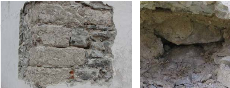
Figure 5: Surface and in-depth probing of the walls.
