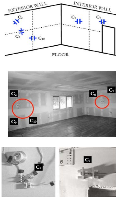
Figure 2: Context and details of instrumentation: top - illustration of crack gauges spanning joints and cracks: mid - photograph of the instrumented room: bottom - details of velocity transducers and crack gauges.
