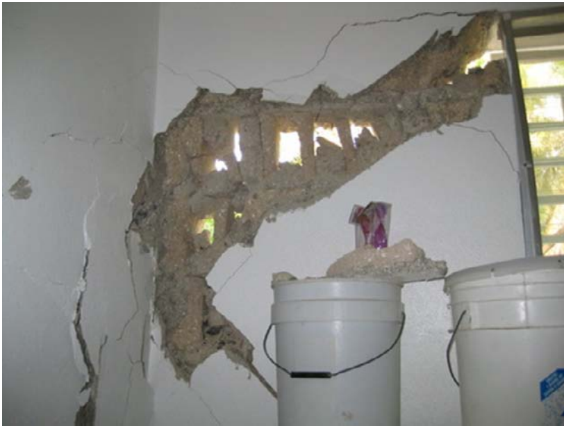
Figure 4: Newly constructed building with a hybrid system of reinforced concrete with CMU block.
