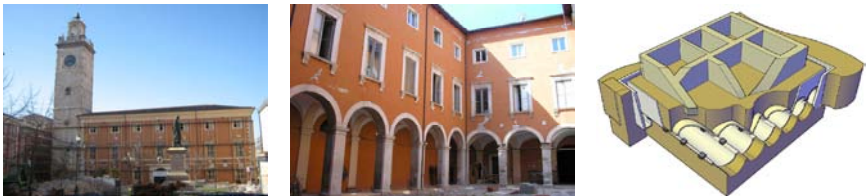
Figure 9: The monumental building Palazzo Margherita in L’Aquila put in safe conditions after of the damages suffered during the 2009 Abruzzo earthquake (left and at the centre); this and further monumental buildings in L’Aquila (including the renowned De Amicis school) may be retrofitted by sub-founding them and inserting a SI system in the sub-foundations, in order to respect the severe conservation requirements applicable in Italy to cultural heritage (among the sub-foundation techniques, that shown on the right, patented by ENEA and the Polytechnic of Torino in 2010, should be used [4]).
