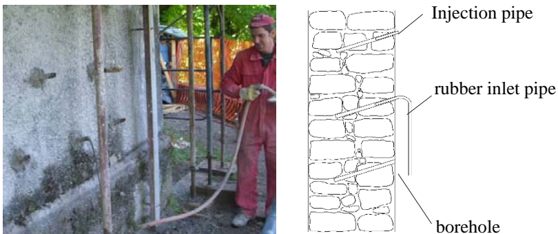
Figure 12: Injection grouting.
