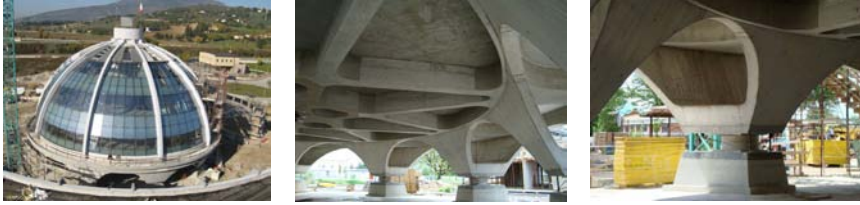
Figure 2: The main building, erected on 10 HDRBs of 1 m diameter (shown at the centre and on the right, covered by provisional protections) and the adjacent service building, isolated by means of HDRBs and SDs, of the Emergency and Management Operative Centre of the new Civil Defence Centre of Central Italy in Foligno, near Perugia (their construction was completed in 2010 and its safety was certified by A. Martelli in February 2011 [3, 4, 7]).
