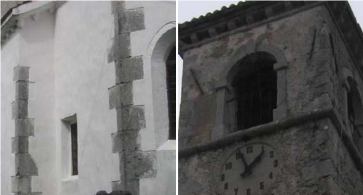
Figure 1: Sewn corners of a St. Michael church in Ljubinj and iron wall ties of the church of St. Andrew in Svino.
