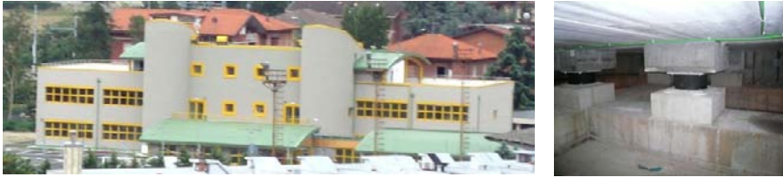
Figure 3: The new school of Marzabotto (Bologna, seismic zone 3), which was isolated (with the collaboration of ENEA) by means of 28 HDRBs and 14 SDs, with 500 mm diameters (it is the first isolated school in Northern Italy; its safety was certified by A. Martelli in September 2010).
