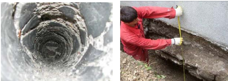
Figure 6: Coring of the walls and in-depth probing of foundations.
