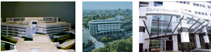
Figure 10: The isolated Nuevo Hospital Militar La Reina in Santiago (Chile), which survived undamaged the Maule earthquake of February 27, 2010 (left), and the isolated Christchurch Woman's Hospital (New Zealand), which had the same behaviour during the event of Canterbury on September 3, 2010 and that of Christchurch on February 21, 2011 (at the centre and right).
