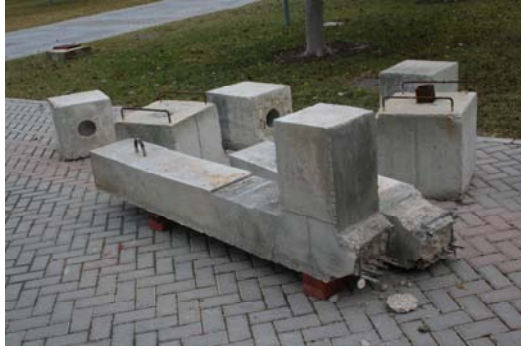
Figure 7: Photograph of the ultimate rupture of prototype 3.
